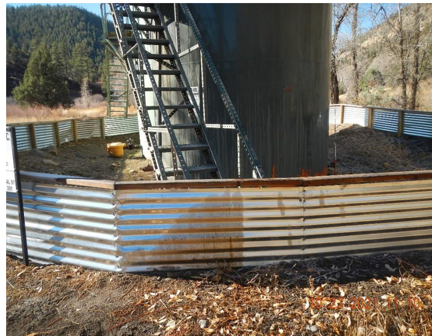
ASTs have been connected to anchors with steel cable.
