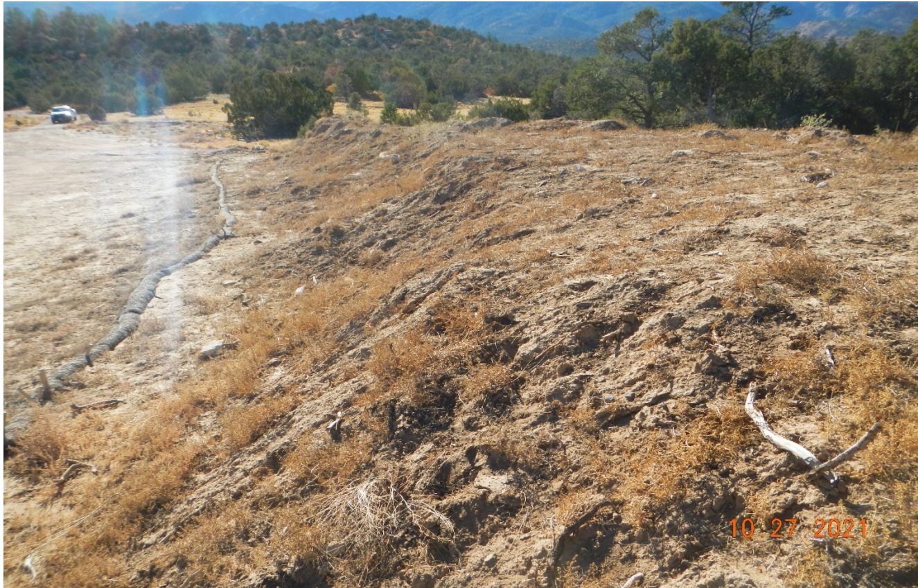
Photo 13. Facing southeast toward the topsoil pile which are not maintained and protected from degradation and weed infestation. Previous corrective action has not been performed. The BMP's around the stockpile are not maintained.
