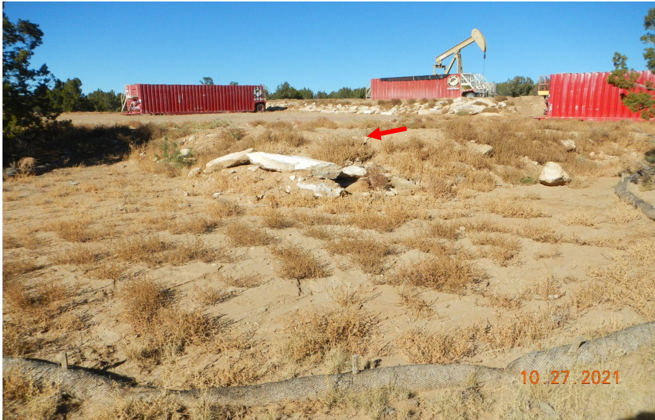
Photo 5. Facing north at the south corner of the location. There is erosion occurring from the disturbed pad site which is filling in the perimeter wattles. Previous corrective action has not been performed.
