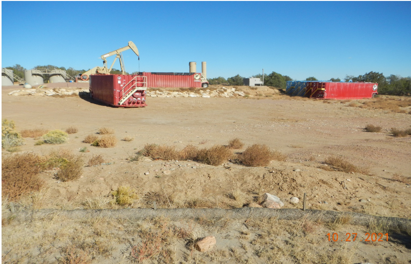
Photo 14. Facing northeast toward the location. The unused tanks need to be removed. Unused areas of the location need to be recontoured and reclaimed. Previous corrective actions have not been performed.
