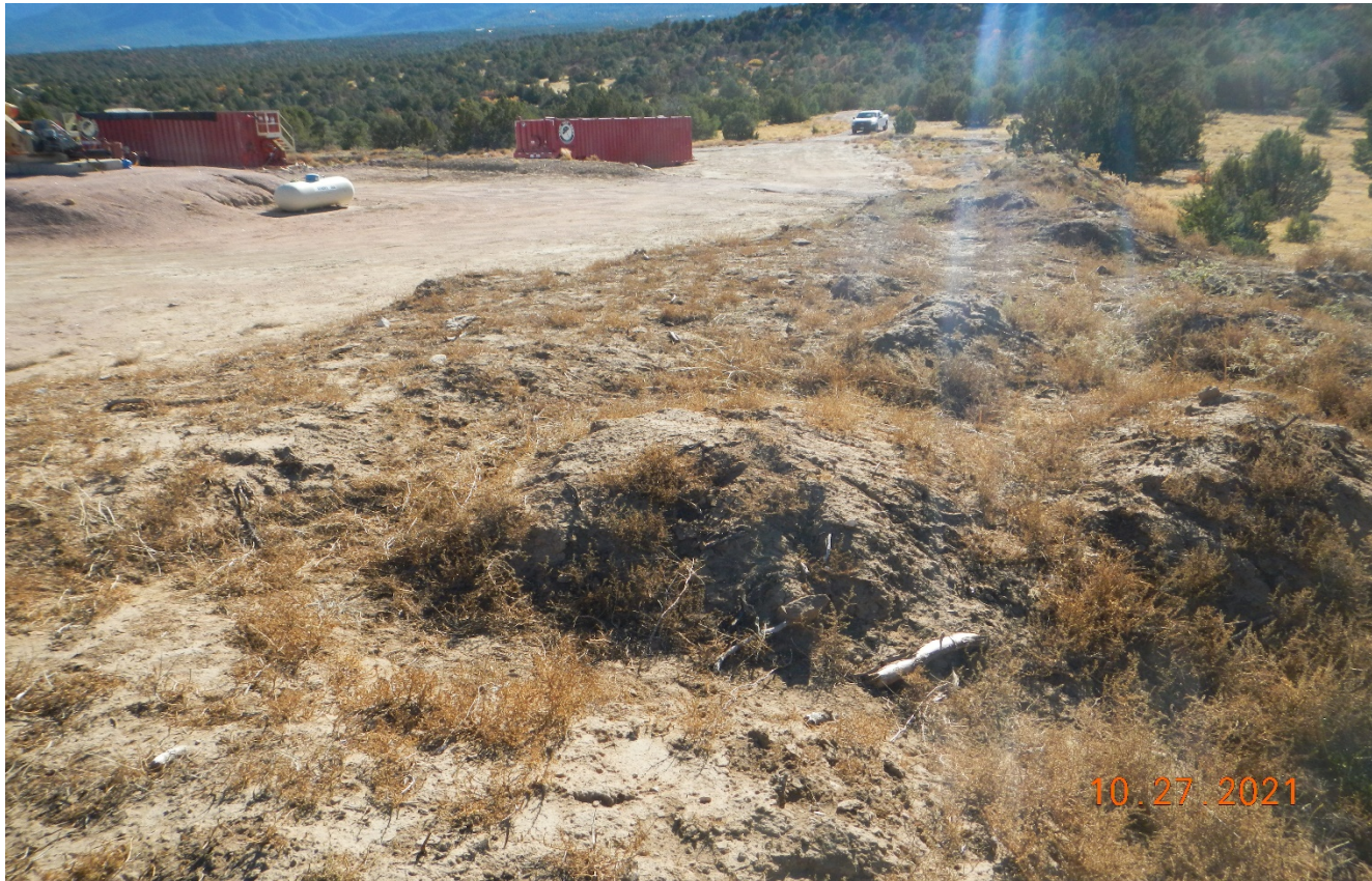
Photo 12. Facing toward the topsoil pile. The topsoil piles are not stabilized and protected. Topsoil piles have not been replaced for interim reclamation. There are undesirable weeds throughout the stockpiles.
