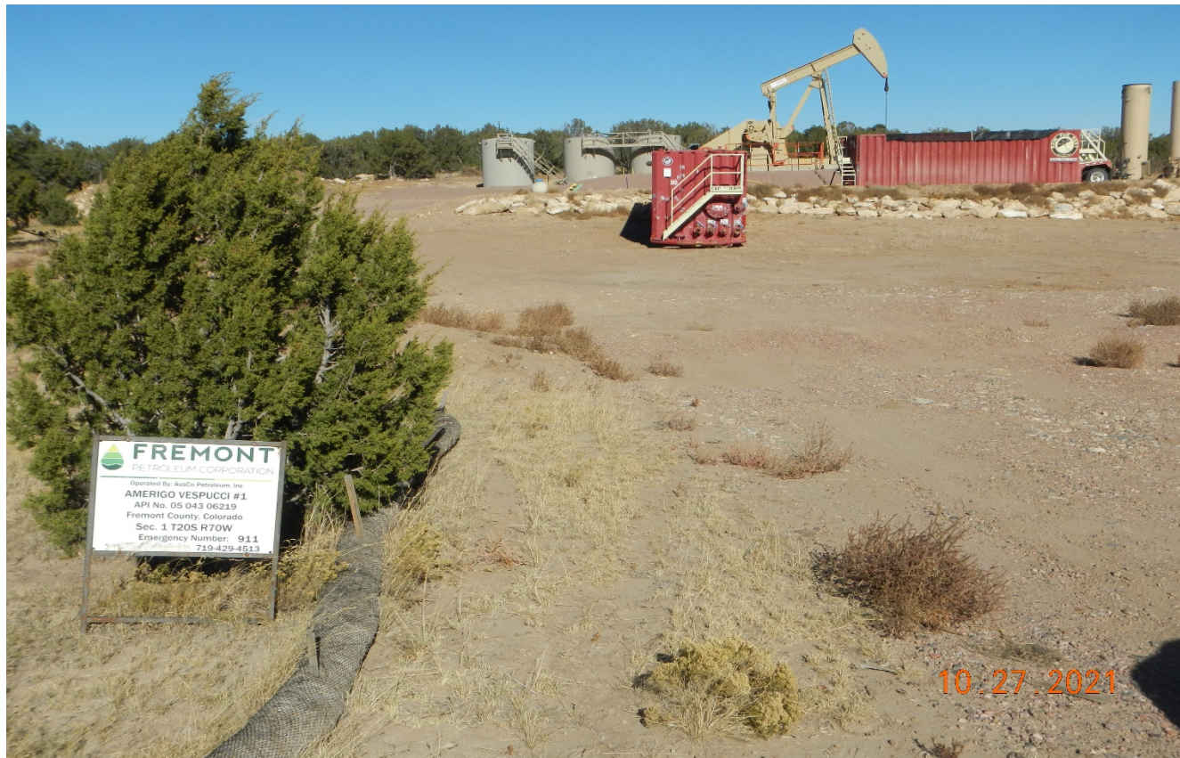
Photo 3. Facing northeast toward the location. Unused equipment has not been removed and interim reclamation has not been performed.
