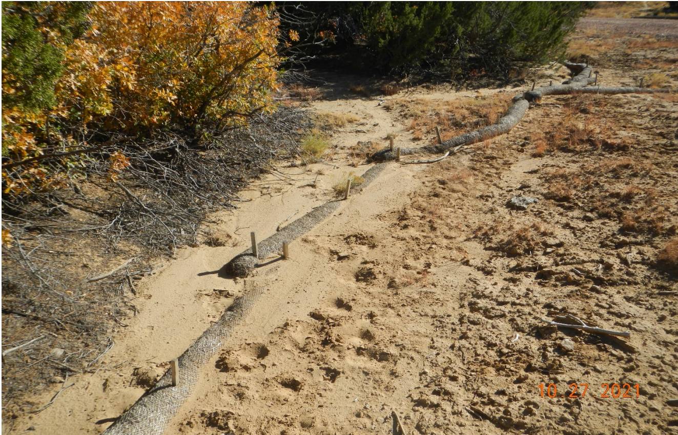
Photo 2. There are wattles along the access road that are filled in with sediment and not maintained.
