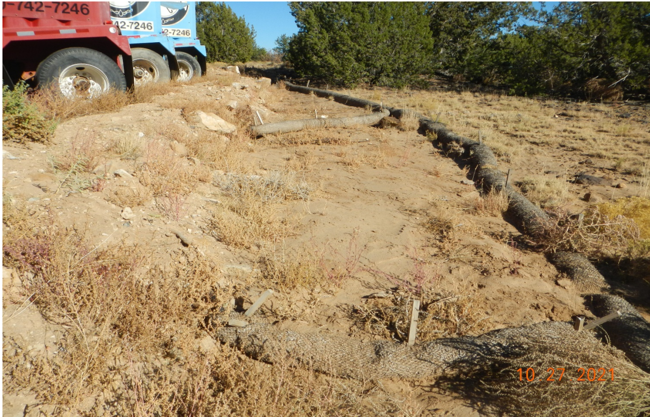
Photo 6. Facing southwest behind the frac tanks. The wattles have filled in with sediment. Previous corrective action has not been performed.
