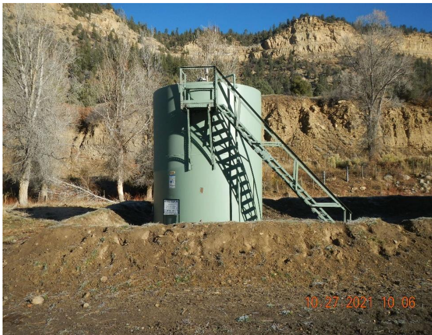
Nielson #4 AST. Uncompacted earthen berm around tank battery.
