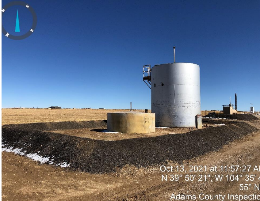
Photo #1 Tanks, separator and meter run.
