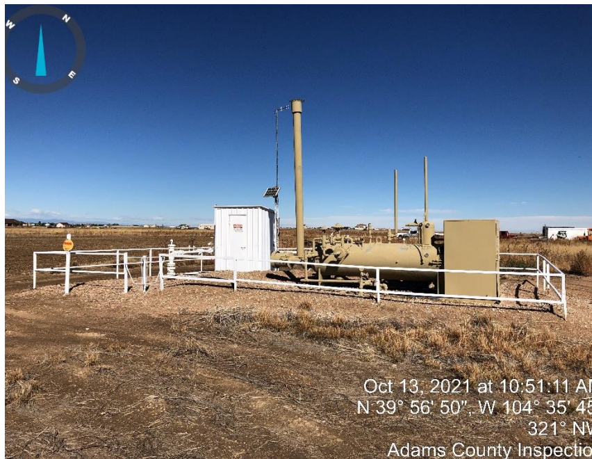
Photo #3 Meter run & Separator.
