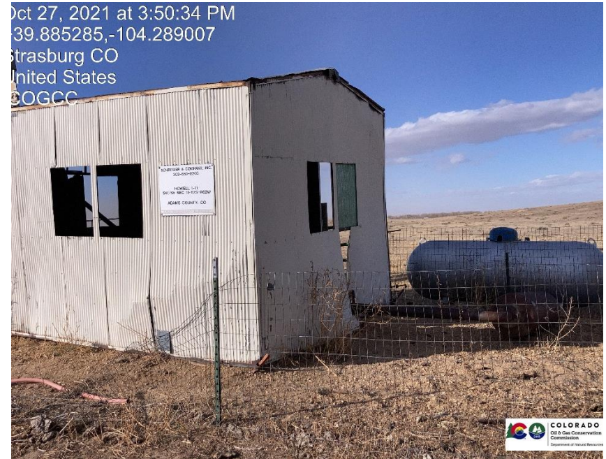
Pic 2 pumpjack house, propane tank needs to be removed.
