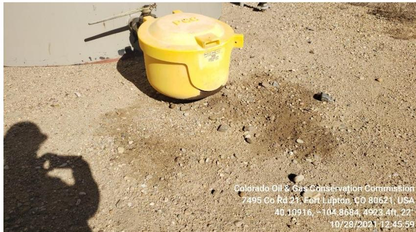
Photo 7 TB placard missing from crude tank
