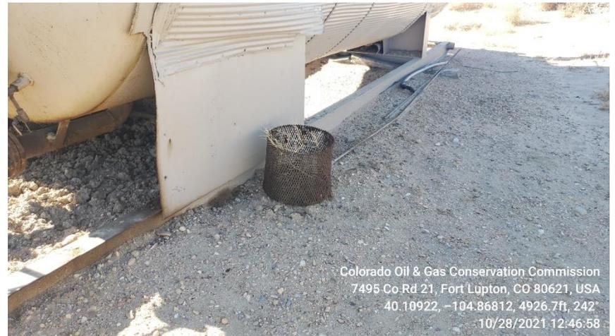
**Photo 9 Bird protector missing from Heater Treater stack**
