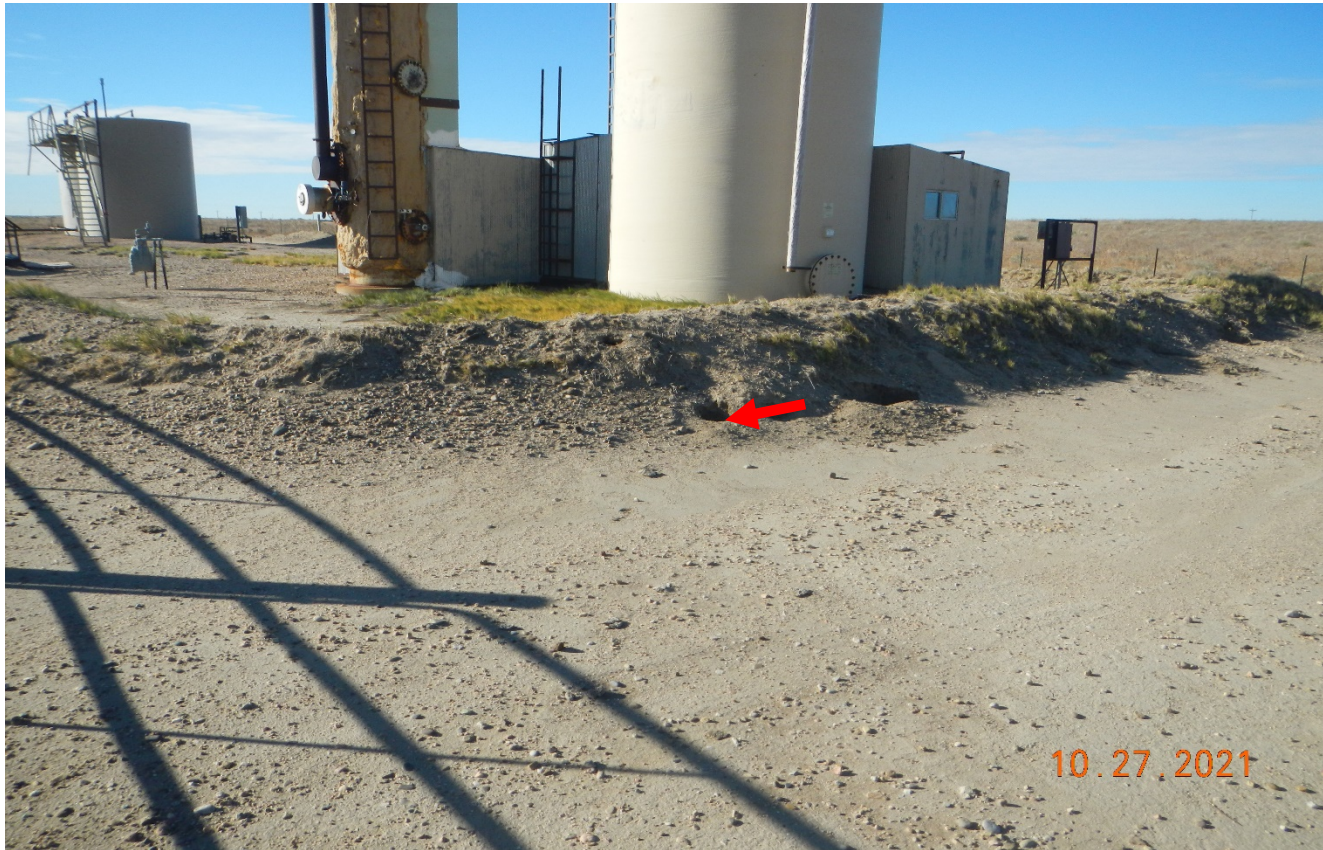
Photo 2. There is animal burrows compromising the berm around the tank battery. The secondary containment is not sufficiently impervious to contain spill. Earthen berms need to be repaired and compacted.
