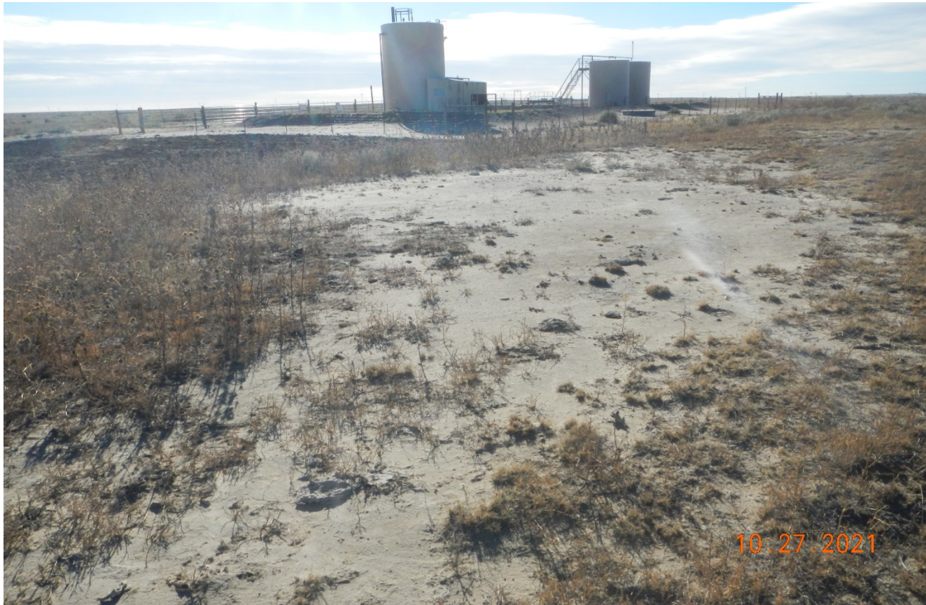
Photo 5. Facing southeast downhill from the tank battery. A former spill had occurred in this area as shown by bare soils. The soils in this area need to be sampled to determine impacted soil properties per 915.b.
