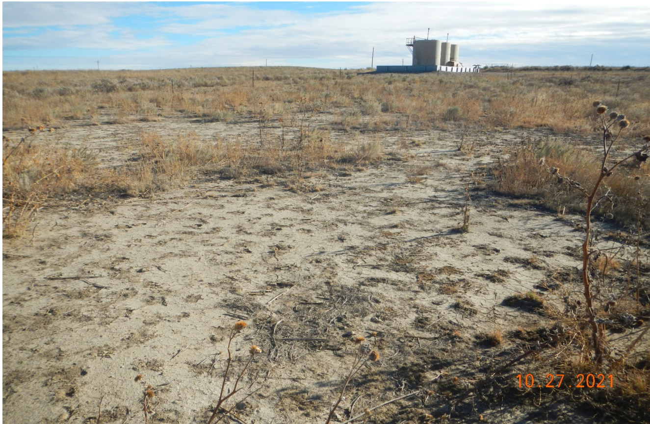
Photo 6. Facing northeast approximately 200' southwest of the tank battery. A former spill had occurred in this area as shown by bare and oil stained soils.
