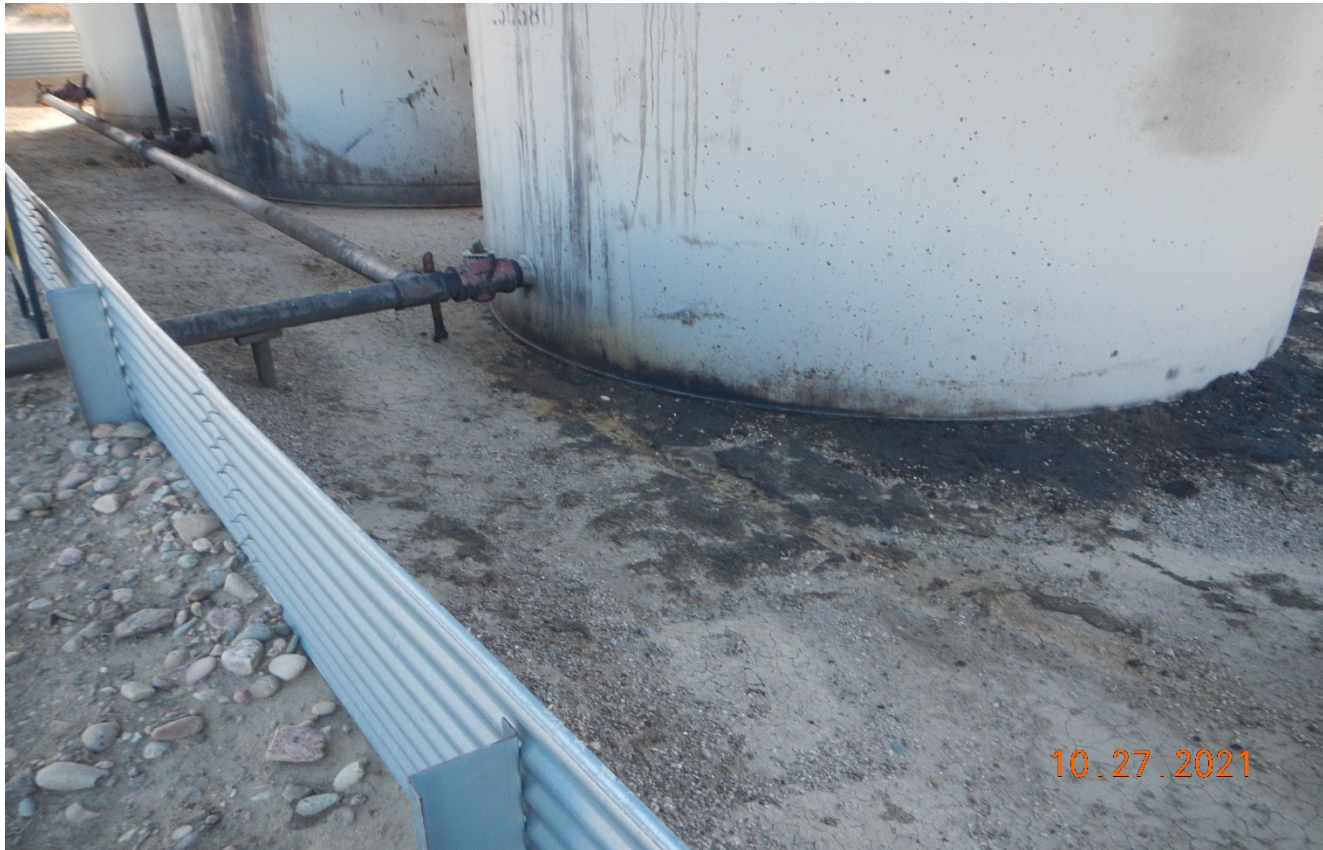
Photo 3. There is oil stained soil around the tanks which need to be cleaned up.
