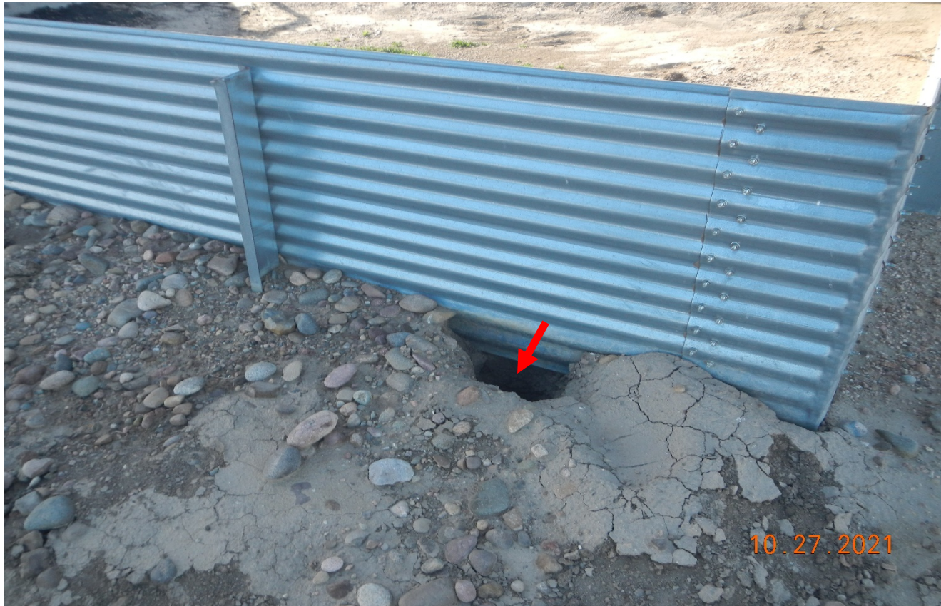
Photo 4. There is a hole at the outside edge compromising the secondary containment of the tank battery.
