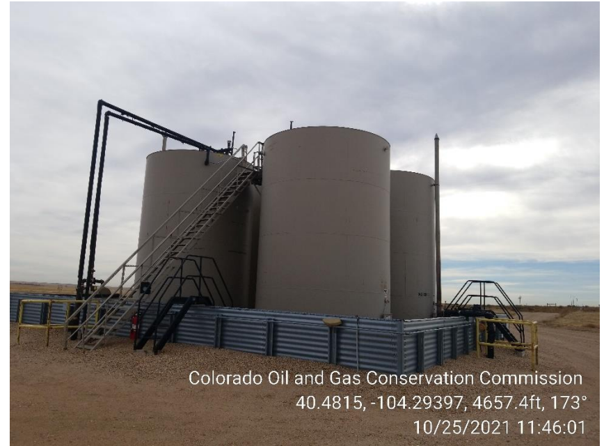
Photo 6 – Tank Battery
