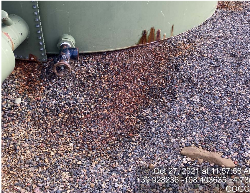
Tank is rusted out and leaking
