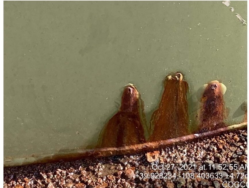
Tank is rusted out and leaking
