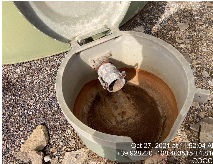
Load out line missing cap/bull plug
