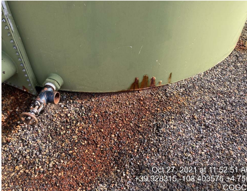
Tank is rusted out and leaking
