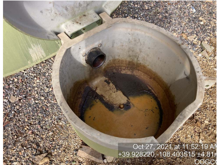
Load out line missing cap/bull plug
