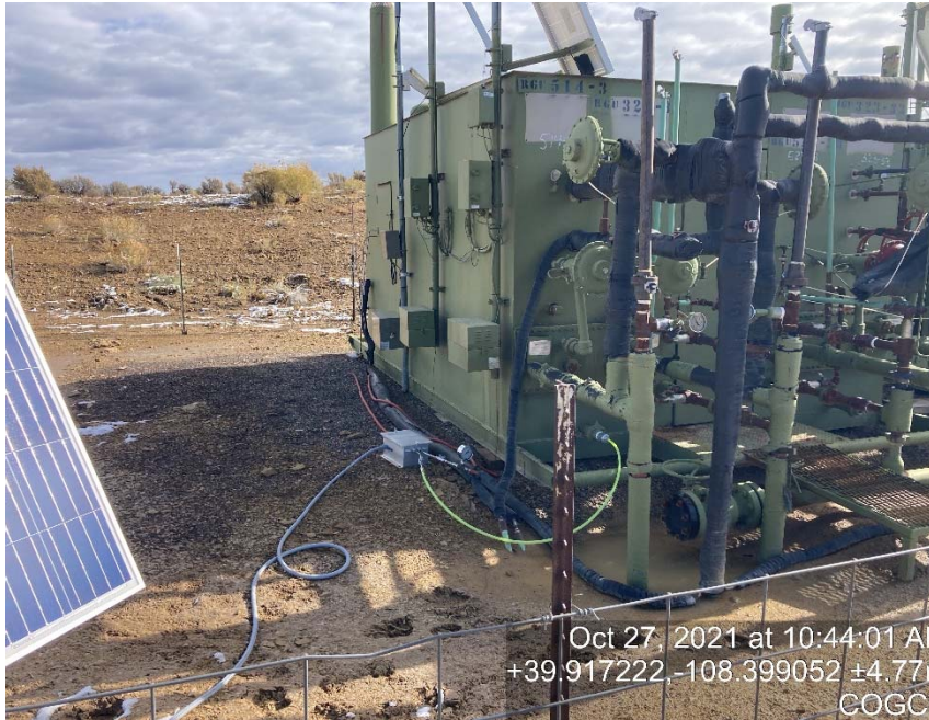
Lack of glycol vessel labeling
