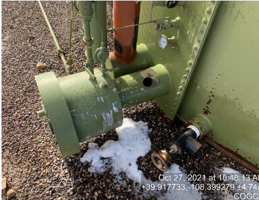
Missing load out cap/bull plug and cap for burner
