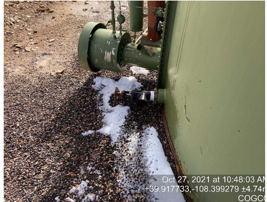
Load out line missing cap/bull plug
