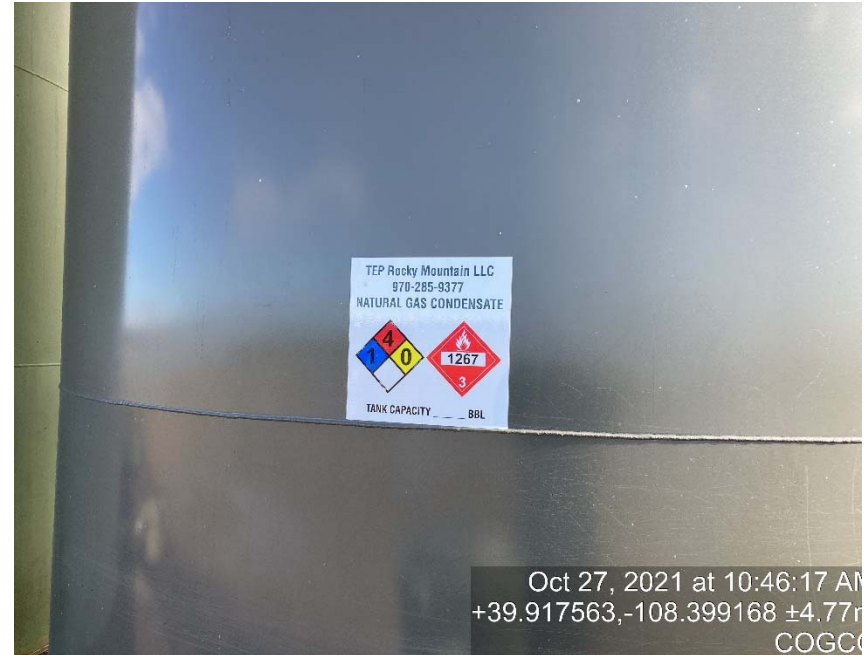
Tank label missing information
