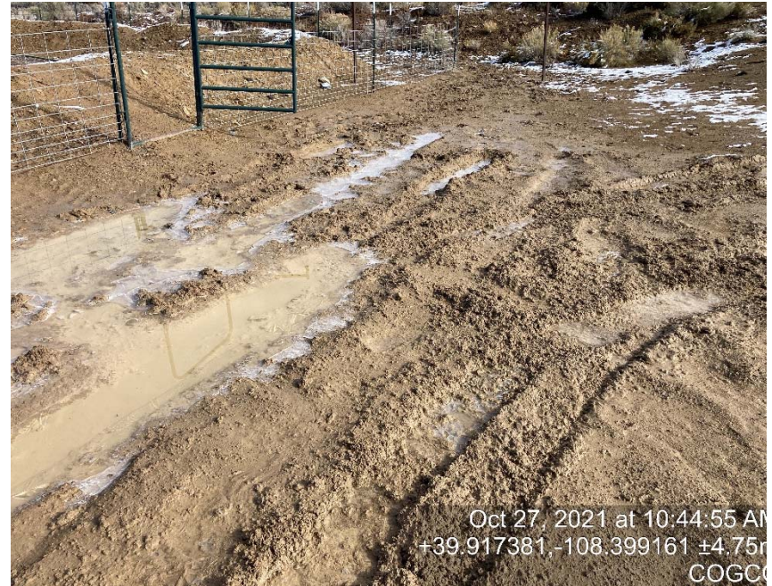
Lack of stabilization/erosion/BMP's failing
