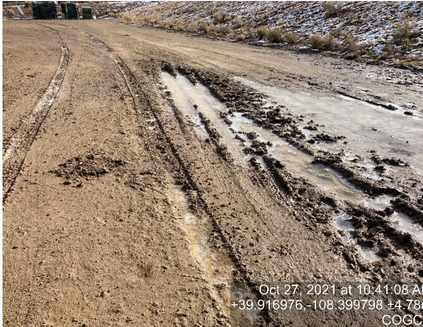
Lack of stabilization/erosion/BMP's failing
