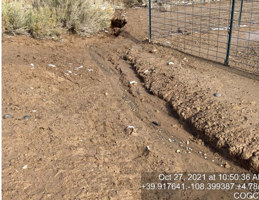
Lack of stabilization/erosion/BMP's failing
