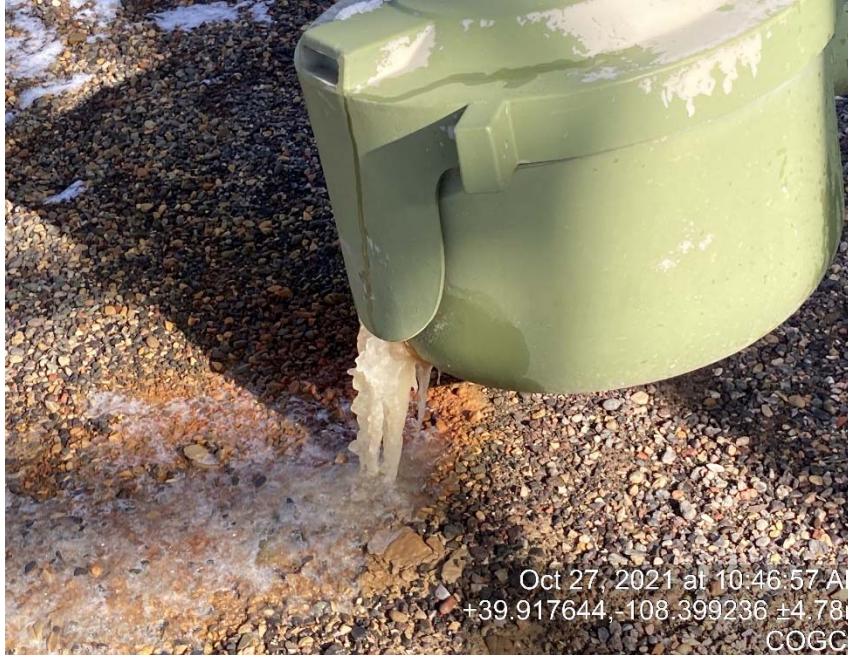
Leaking load out line with out cap/bull plug and staining
