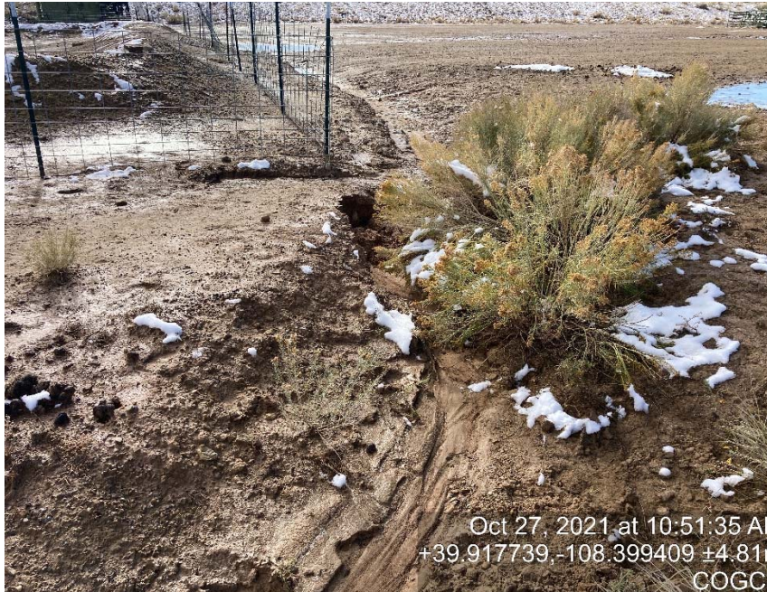
Lack of stabilization/erosion/BMP's failing
