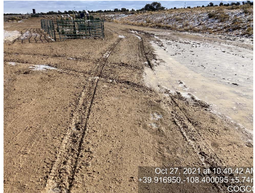
Lack of stabilization/erosion/BMP's failing
