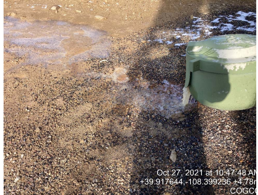
Leaking load out line with out cap/bull plug and staining
