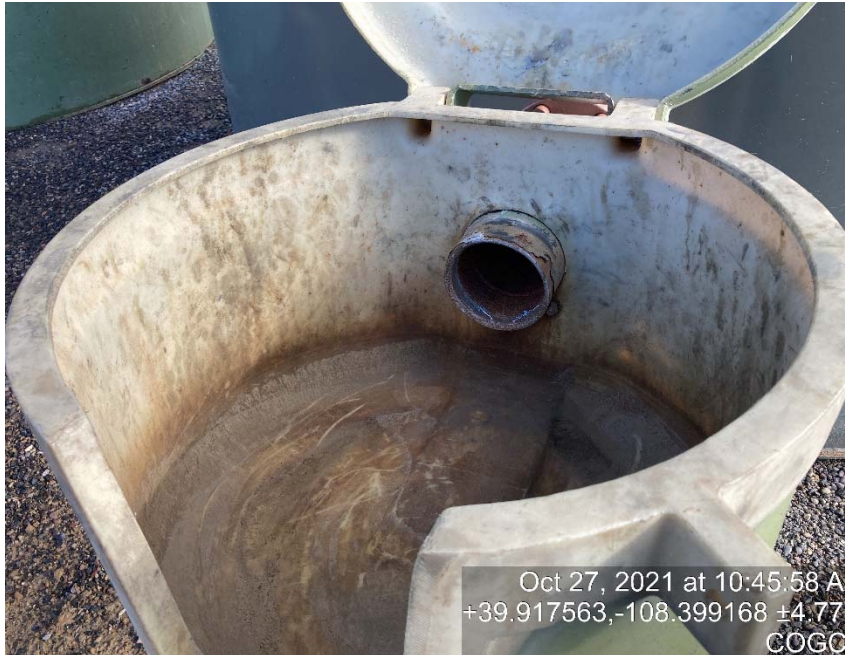
Load out line missing cap/bull plug
