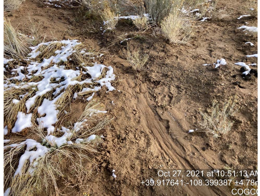
Lack of stabilization/erosion/BMP's failing
