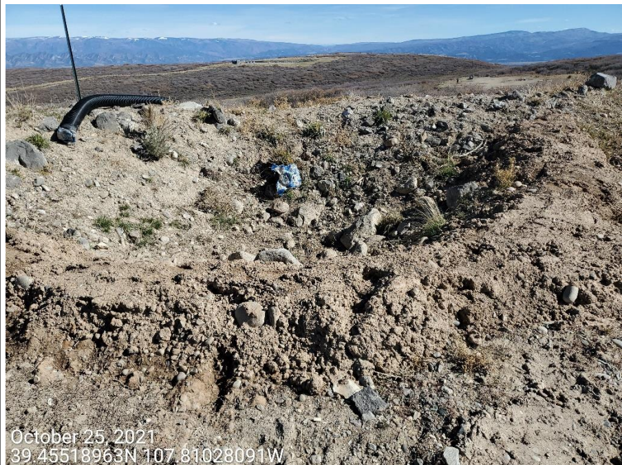
Photo 1: Photos show the sediment traps on the NW/NE corners of the production area. Photos show controls have not been installed in accordance with good engineering practices to allow for proper stormwater discharge.
