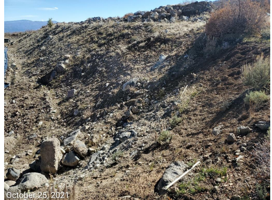
Photo 2: Photos provide examples showing that control measures to protect and stabilize the cut slopes of the Location remain missing or insufficient.
