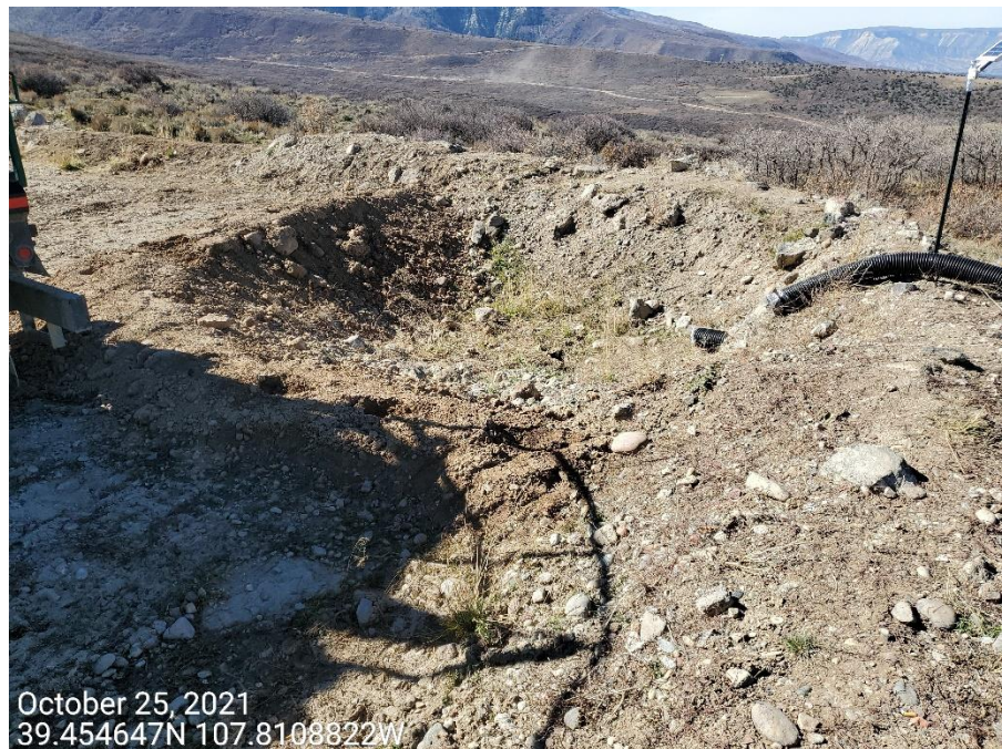
Photo 1: Photos show the sediment traps on the NW/NE corners of the production area. Photos show controls have not been installed in accordance with good engineering practices to allow for proper stormwater discharge.
