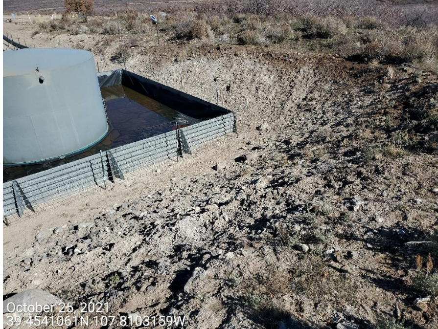
Photo 2: Photos provide examples showing that control measures to protect and stabilize the cut slopes of the Location remain missing or insufficient.
