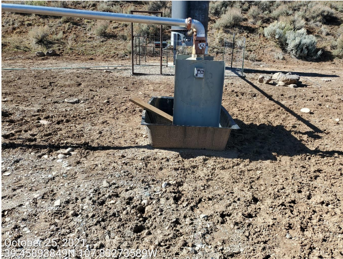
Photo 1: Photo shows that Operator has placed a board into the containment BMPs; control measures to prevent wildlife access to the containment BMP remains inadequate.
