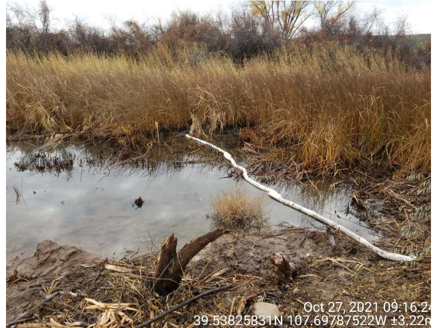
Photo #12 – Absorbent boom installed downstream of reported point of release. Note density of vegetation in wetlands area.
