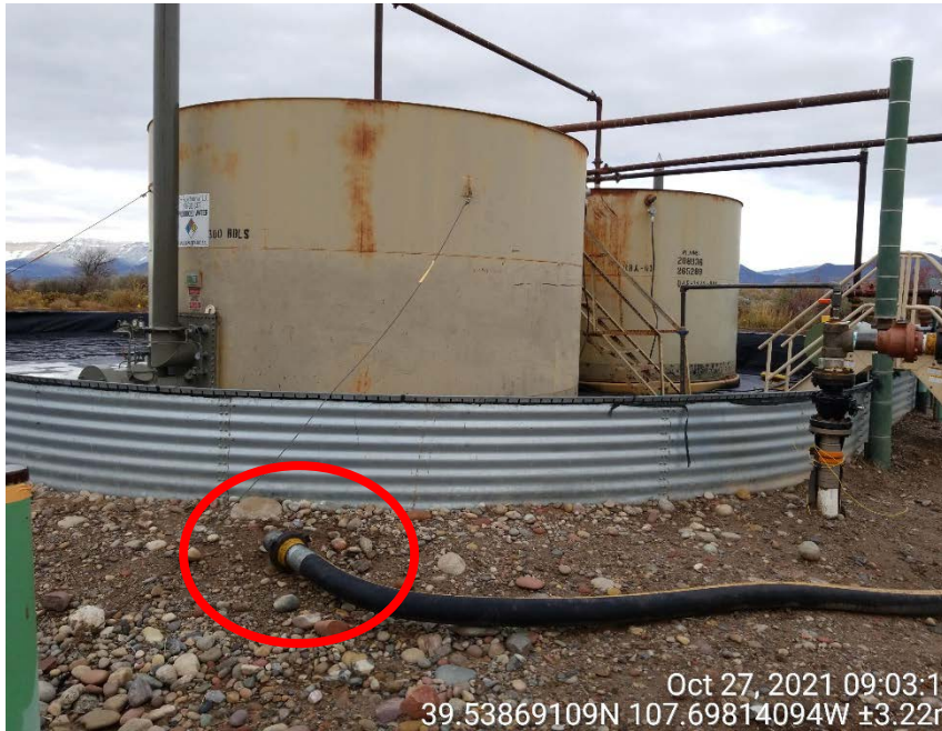
Photo #3 – Tank battery loadout hose stored outside of secondary containment area.
