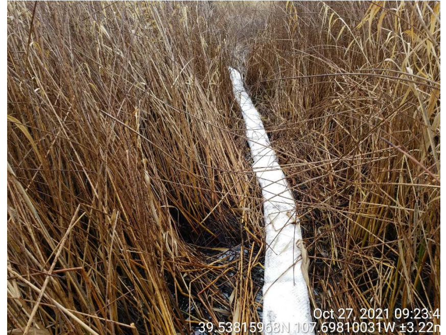
Photo #14 – Additional boom installed across wetlands area downstream from point of release.
