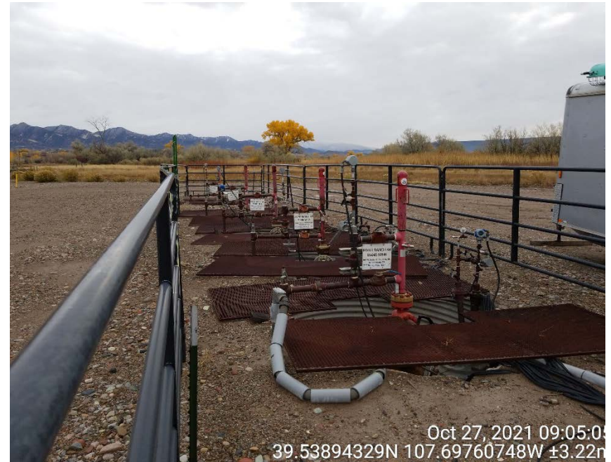
Photo #4 – Overview of wellheads. Well cellars contained fluids on inspection date. Gas bubbles were observed in the cellars for the A1, A4, and A5 wells during inspection.
