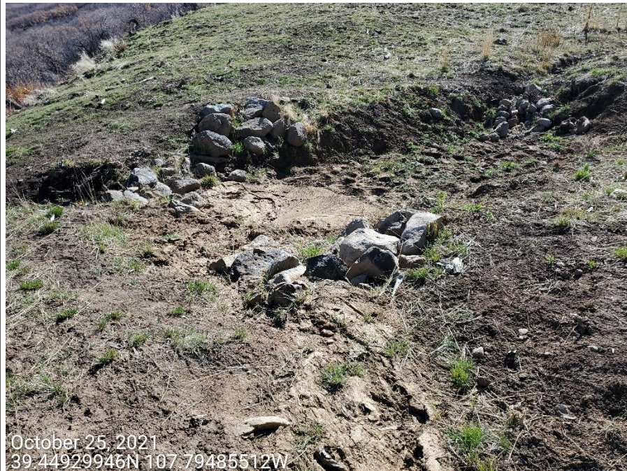
Photo 5: Photos taken from the sediment trap on the east end of the Location. Control has not been constructed with and appropriate inlet/outlet per good engineering practices; geotextile lining not observed; erosion degradation under/around rip-rap material evident (photo right); offsite erosion degradation and sediment transport observed below outlet.
