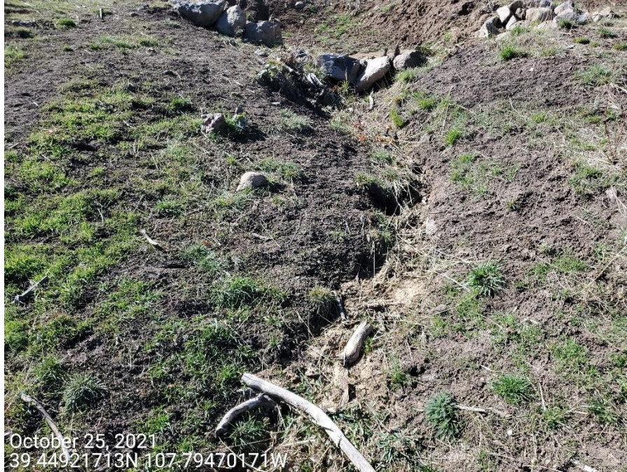
Photo 6. Continued from photo 5. Photo shows stormwater erosion degradation and offsite sediment transport below the sediment trap outlet.
