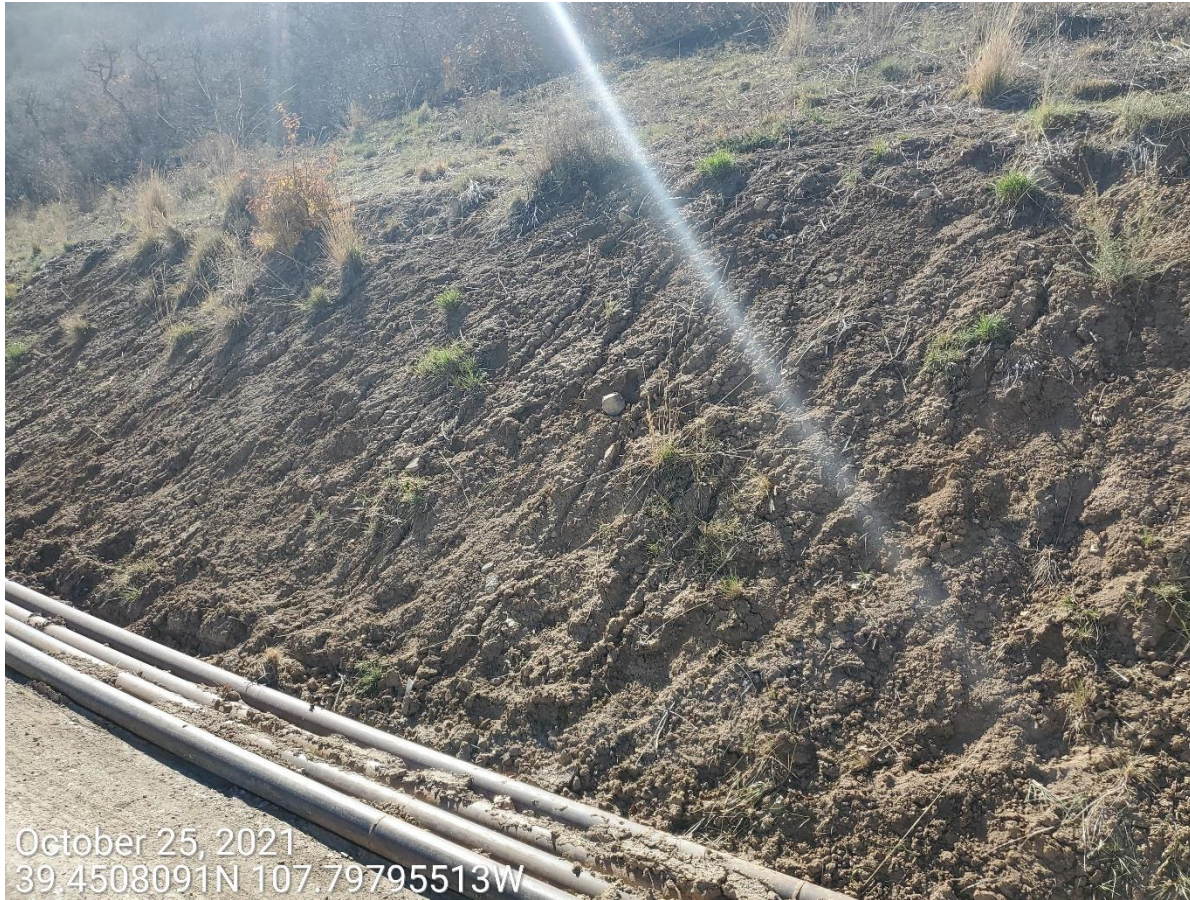
Photo 3.a: Photo shows control measures to protect and stabilize the cut slopes along the access road are missing or insufficient.
