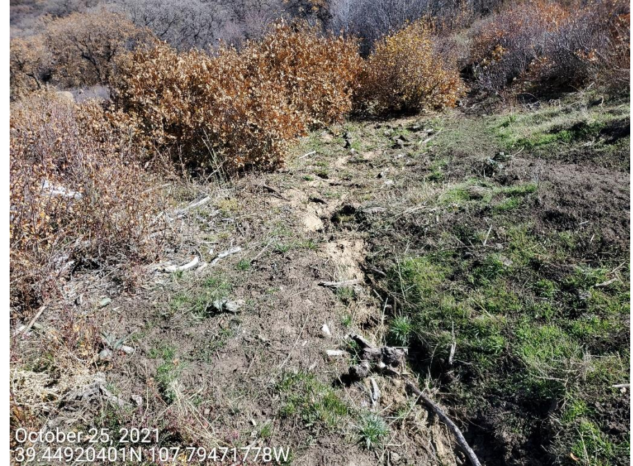
Photo 6. Continued from photo 5. Photo shows stormwater erosion degradation and offsite sediment transport below the sediment trap outlet.
