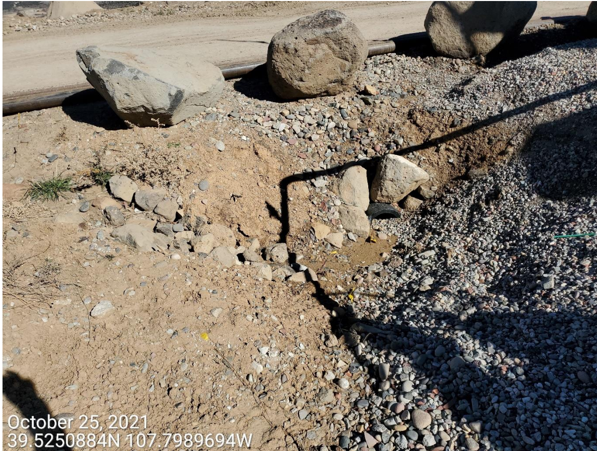
Photo 14: Photo shows culvert at the Location entrance has filled with sediment.
