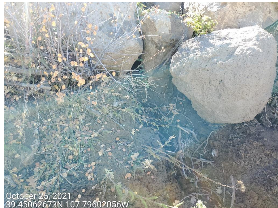
Photo 4: Photos taken from the sediment trap at the Location entrance (west end of the Location). Control has not been constructed with and appropriate inlet/outlet per good engineering practices; geotextile lining not observed; erosion degradation under/around rip-rap material evident (photo right); offsite erosion degradation and sediment transport observed below outlet.
