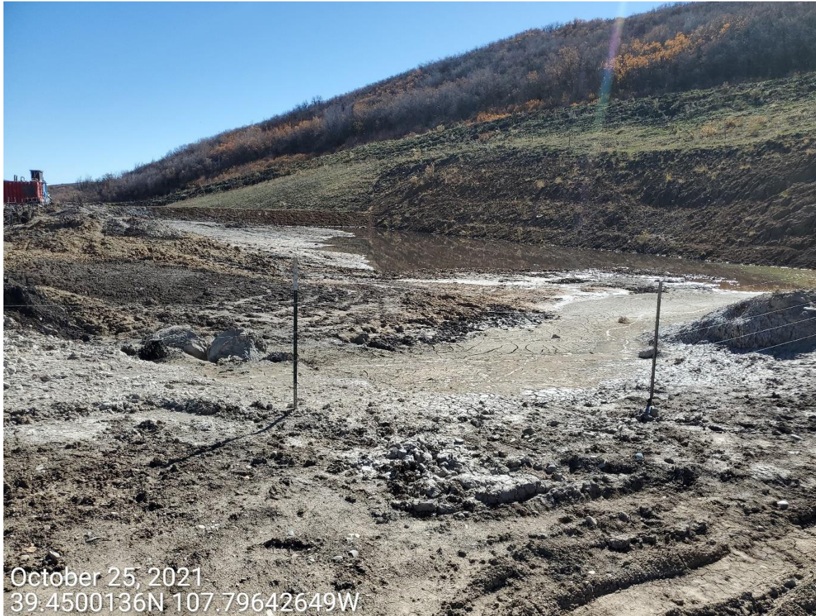
Photo 13: Photo shows the cuttings trench on the southwest end of the Location. Trench/pit requires permitting. Photo also shows that stormwater has been allowed to flow into the cuttings trench and is now considered E&P waste; fluids required removal and disposal.
