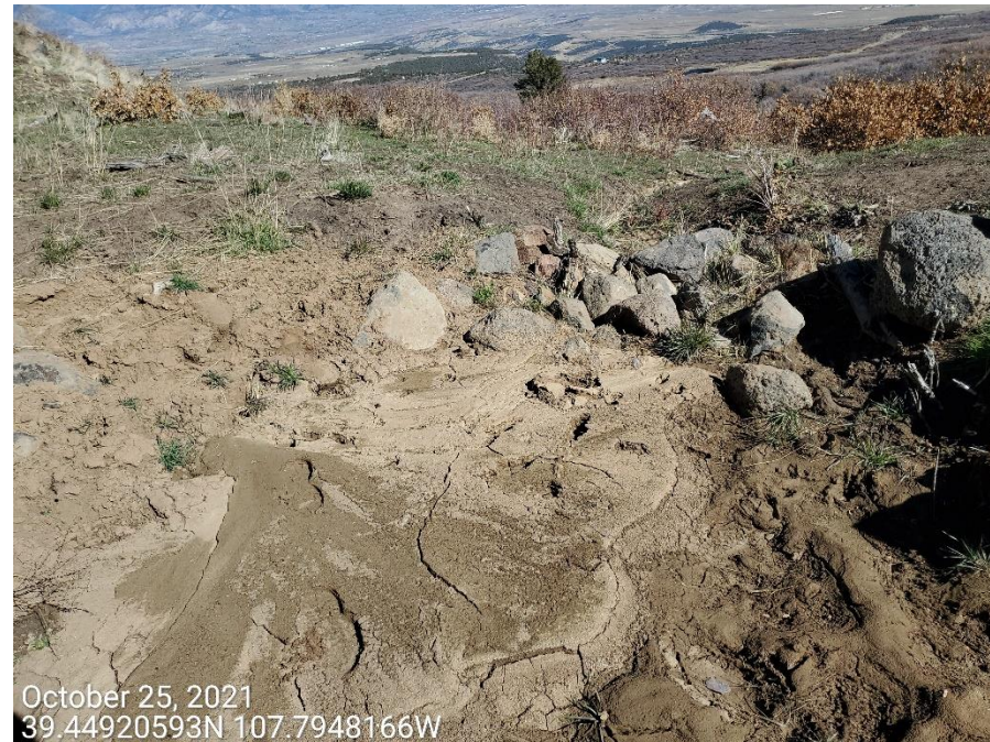
Photo 5: Photos taken from the sediment trap on the east end of the Location. Control has not been constructed with and appropriate inlet/outlet per good engineering practices; geotextile lining not observed; erosion degradation under/around rip-rap material evident (photo right); offsite erosion degradation and sediment transport observed below outlet.
