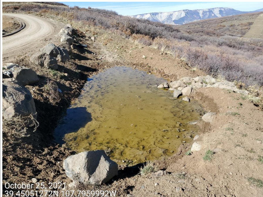
Photo 4: Photos taken from the sediment trap at the Location entrance (west end of the Location). Control has not been constructed with and appropriate inlet/outlet per good engineering practices; geotextile lining not observed; erosion degradation under/around rip-rap material evident (photo right); offsite erosion degradation and sediment transport observed below outlet.
