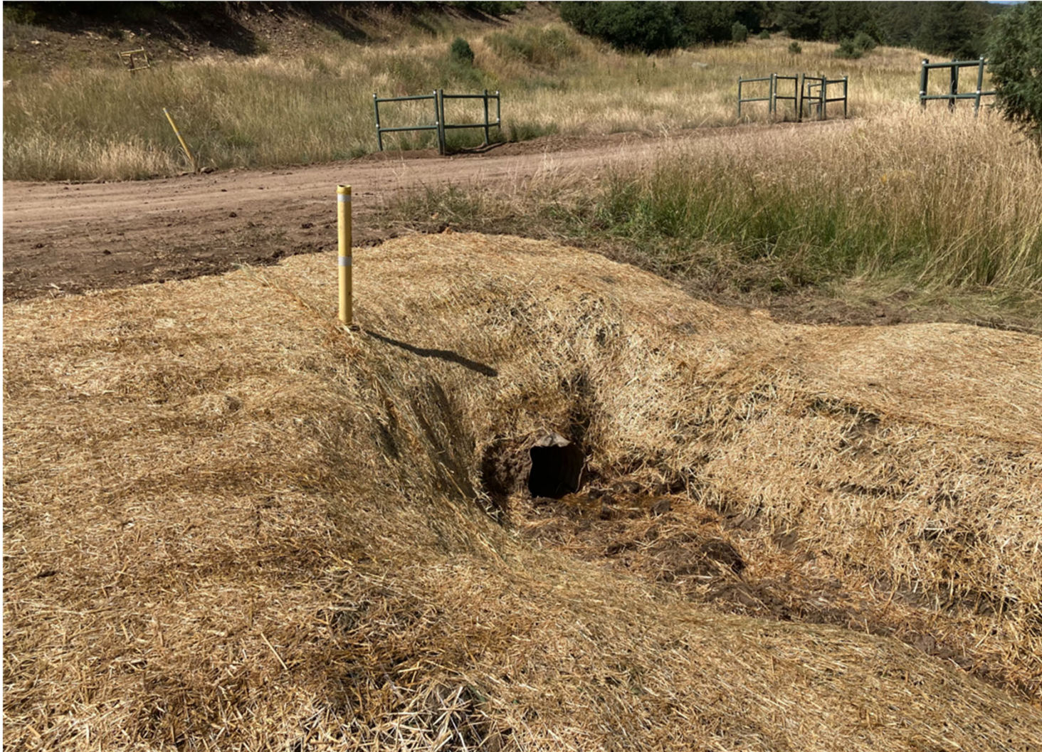
PHOTO 2: THE CULVERT OUTLET ON THE MAIN LEASE ROAD OF BIG BINGHAM CANYON AND THE RIDGE ROAD INTERSECTION WAS BELOW GRADE AND WOULD NOT DRAIN PROPERLY. POSITIVE DRAINAGE WAS ESTABLISHED FOR THE OUTLET. THE DISTURBED SOIL WAS SEEDED WITH AN APPROVED CPW SEED MIX TO ESTABLISH VEGETATION. EROSION CONTROL BLANKETS WERE INSTALLED FOR TEMPORARY SOIL STABILIZATION.
