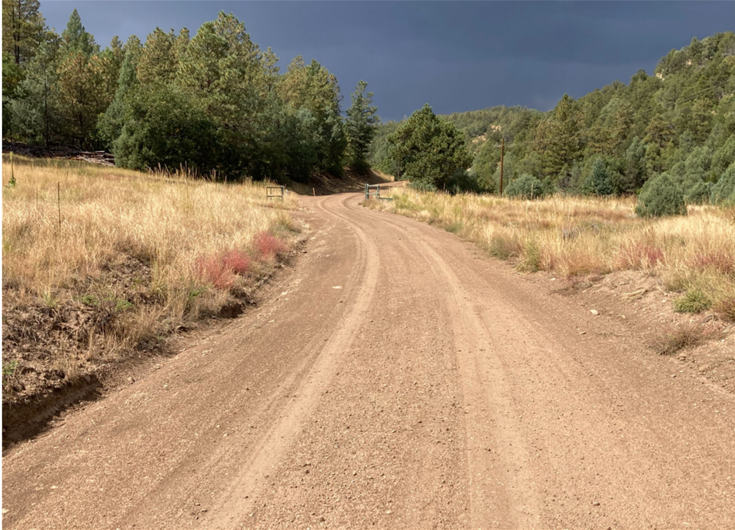
PHOTO 4: THE ROAD SURFACE WAS CROWNED TO CREATE SHEET FLOW AND ELIMINATE THE TIRE RUTS. ADDITIONAL GRAVEL WAS INSTALLED TO THE ROADWAY SURFACE TO IMPROVE STABILIZATION EFFORTS.
