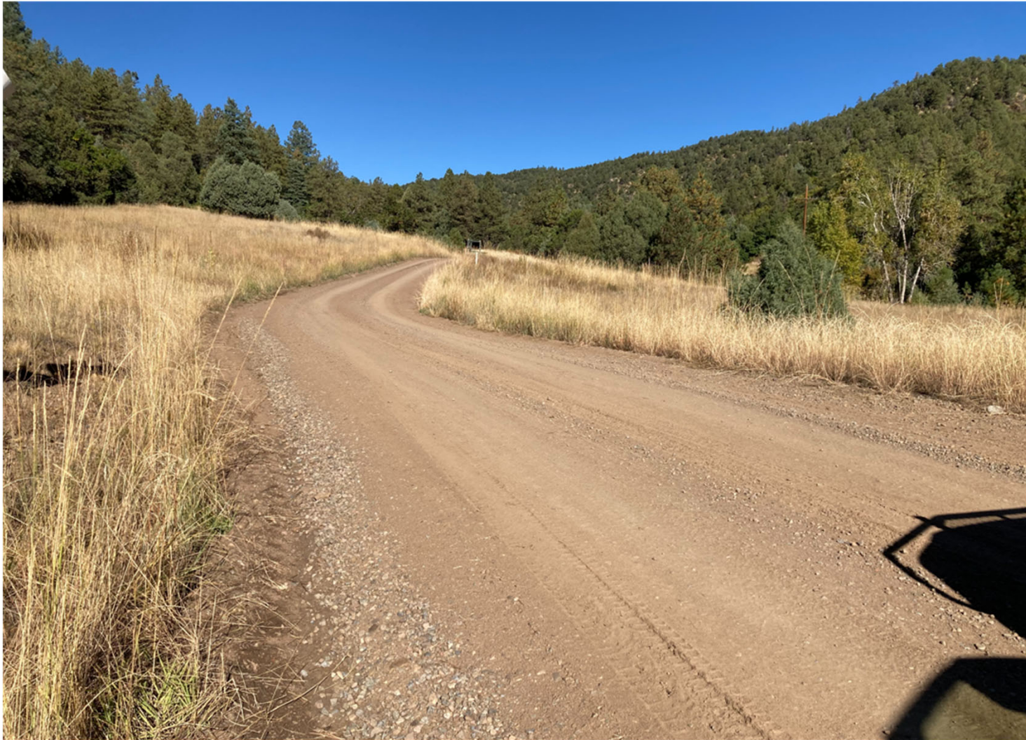
PHOTO 3: THE ROAD SURFACE WAS CROWNED TO CREATE SHEET FLOW AND ELIMINATE THE TIRE RUTS. ADDITIONAL GRAVEL WAS INSTALLED TO THE ROADWAY SURFACE TO IMPROVE STABILIZATION EFFORTS.
