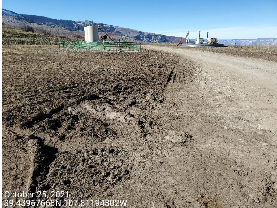
Photo 1: Photos show control measures to stabilize the production areas of the Location, and to mitigate tracking and offsite sediment transport have not been maintained in proper functioning condition, and are now inadequate.
