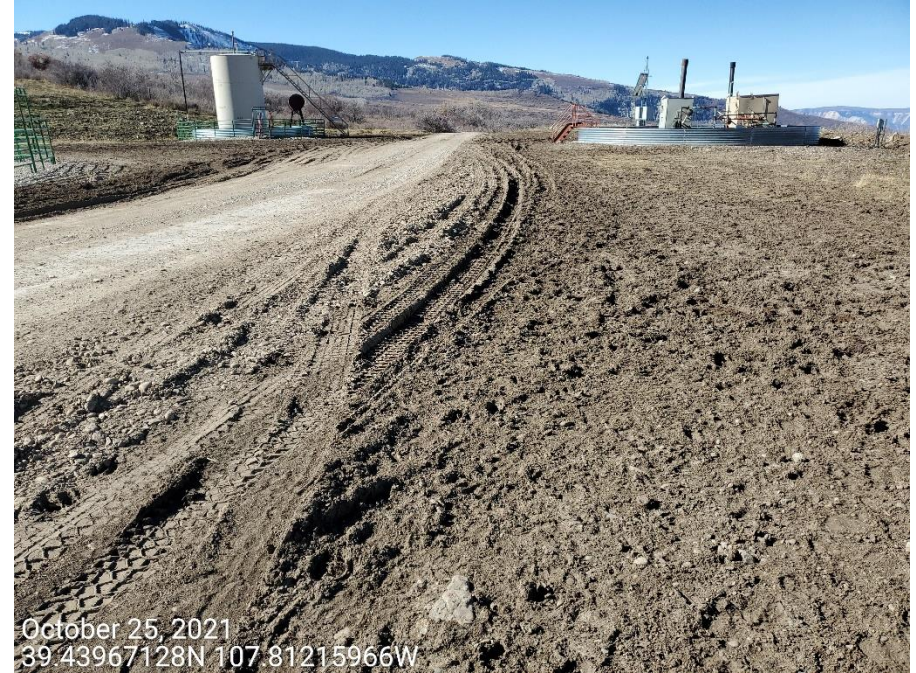
Photo 1: Photos show control measures to stabilize the production areas of the Location, and to mitigate tracking and offsite sediment transport have not been maintained in proper functioning condition, and are now inadequate.
