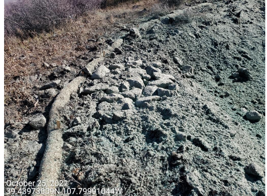
Photo 8: Photos examples showing the sediment traps on the northwest end of the Location. Sediment trap control measures remain unchanged since previous inspection. It is unclear if traps are appropriate in size to manage runoff from the drainage area of the pad and upslope undisturbed areas. Geotextile lining not observed at inlet/outlet.
