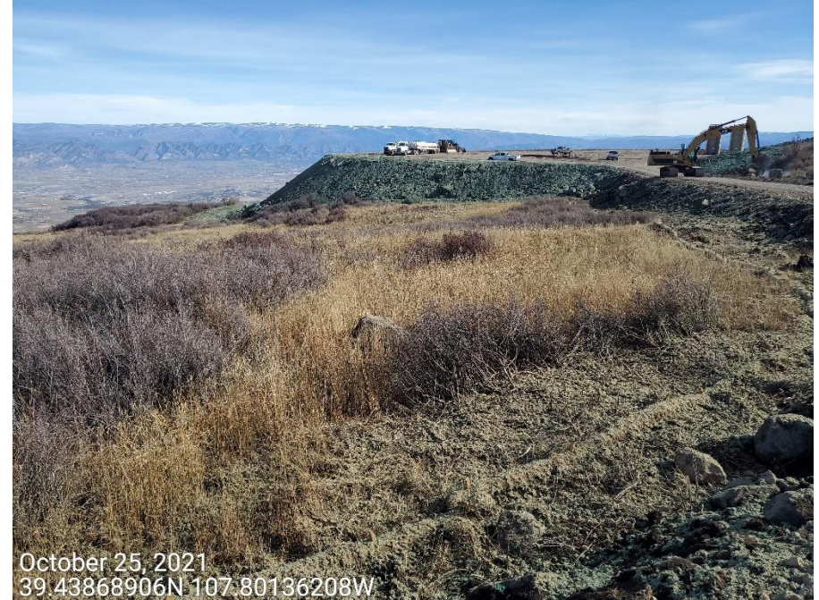
Photo 5: Photos examples showing Operator has implemented a hydro mulch on the cut/fill slopes, and the soil stockpile.
