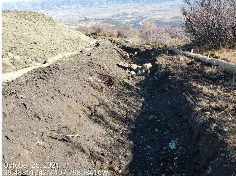
Photo 6. Photos taken from the perimeter stormwater diversion ditch. Photos show that the stormwater diversion ditch has not been constructed in accordance with good engineering practices, and remain improperly constructed with vertical slopes and unconsolidated soils.
