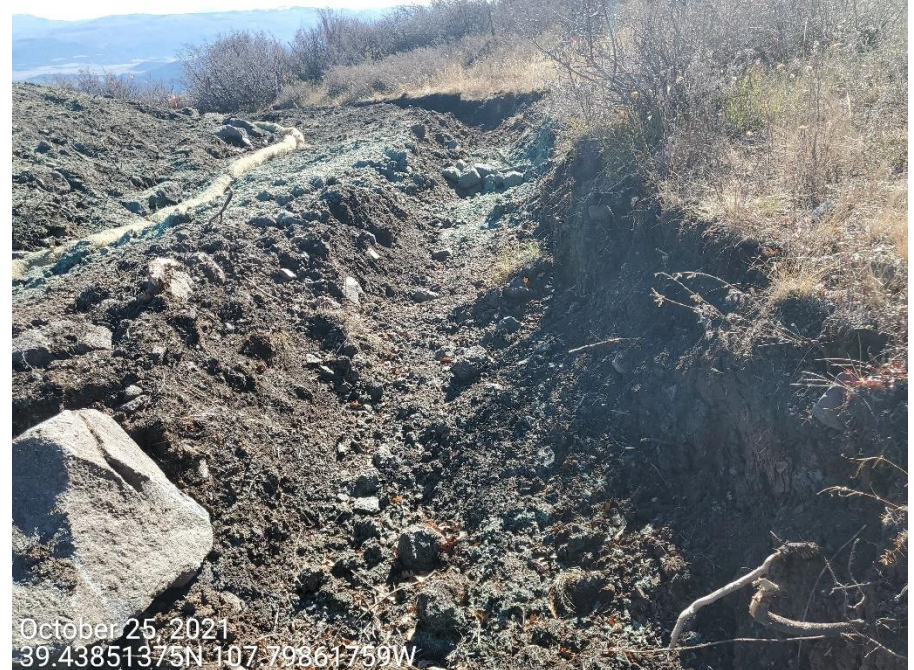
Photo 6. Photos taken from the perimeter stormwater diversion ditch. Photos show that the stormwater diversion ditch has not been constructed in accordance with good engineering practices, and remain improperly constructed with vertical slopes and unconsolidated soils.
