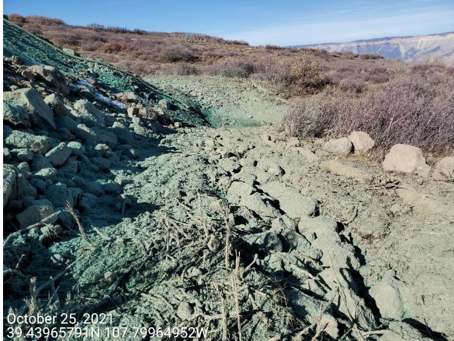
Photo 8: Photos examples showing the sediment traps on the northwest end of the Location. Sediment trap control measures remain unchanged since previous inspection. It is unclear if traps are appropriate in size to manage runoff from the drainage area of the pad and upslope undisturbed areas. Geotextile lining not observed at inlet/outlet.
