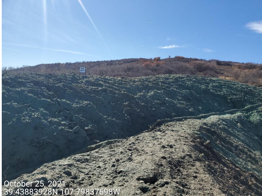
Photo 5: Photos examples showing Operator has implemented a hydro mulch on the cut/fill slopes, and the soil stockpile.
