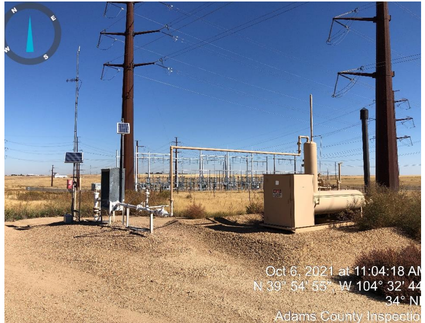
Photo #2 Meter run & Separator.
