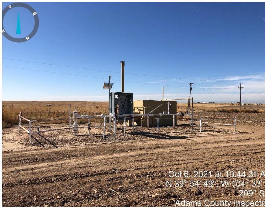
Photo #2 Meter run & Separator.
