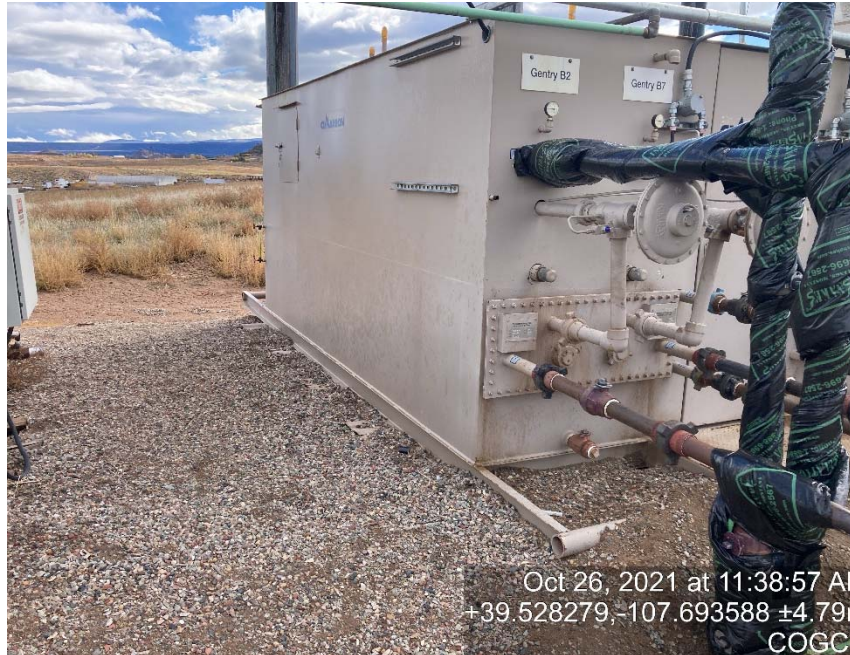
Lack of labeling on glycol storage vessel
