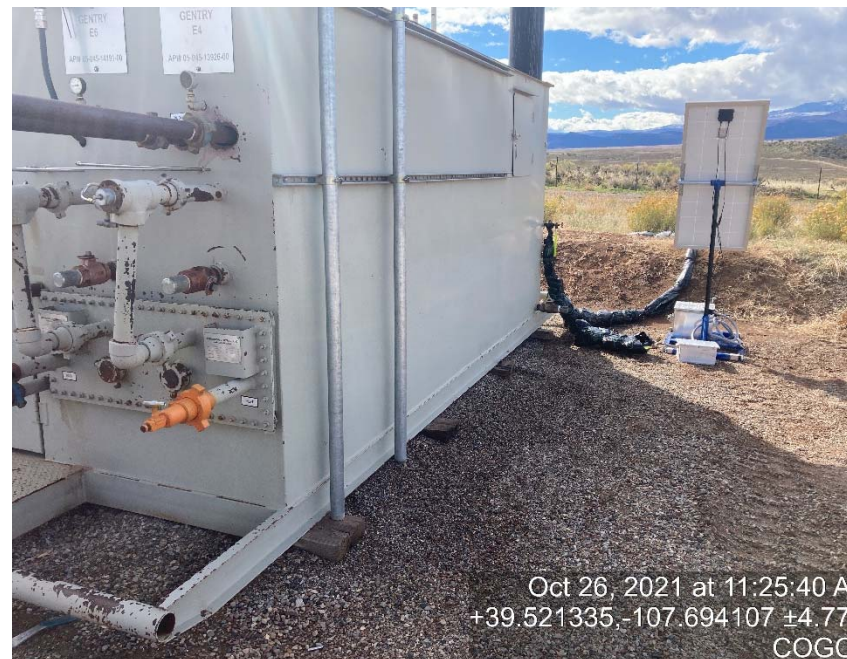
Lack of labeling on glycol storage vessels
