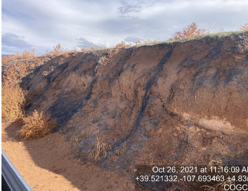
Lack of stabilization/failing BMP's
