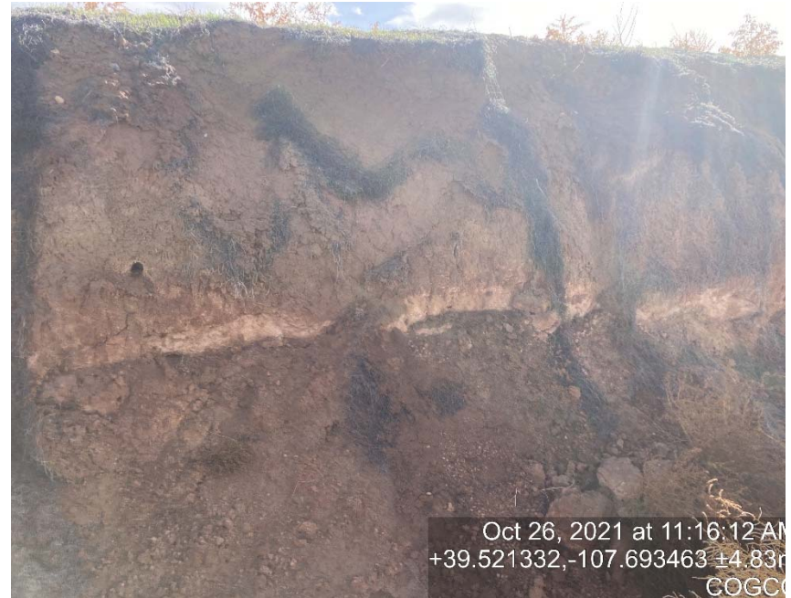
Lack of stabilization/failing BMP's
