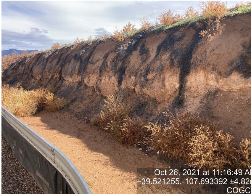
Lack of stabilization/failing BMP's
