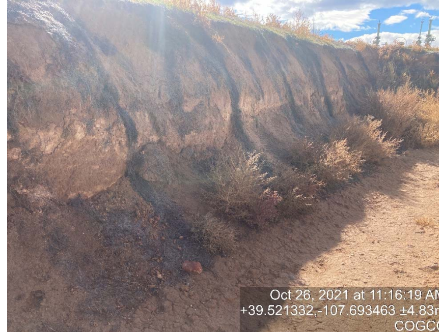
Lack of stabilization/failing BMP's
