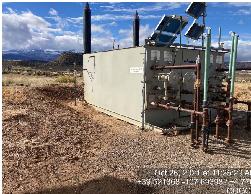
Lack of labeling on glycol storage vessels
