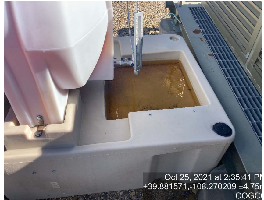
Chemical tank containment is full of fluid
