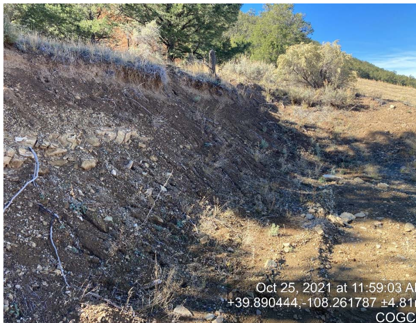
Lack of stabilization/erosion
