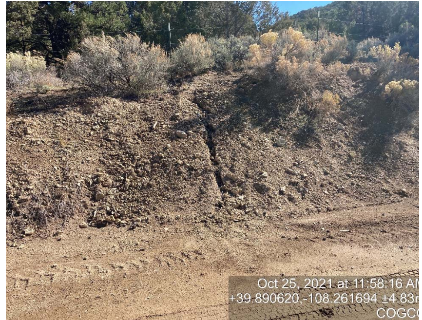
Lack of stabilization/erosion
