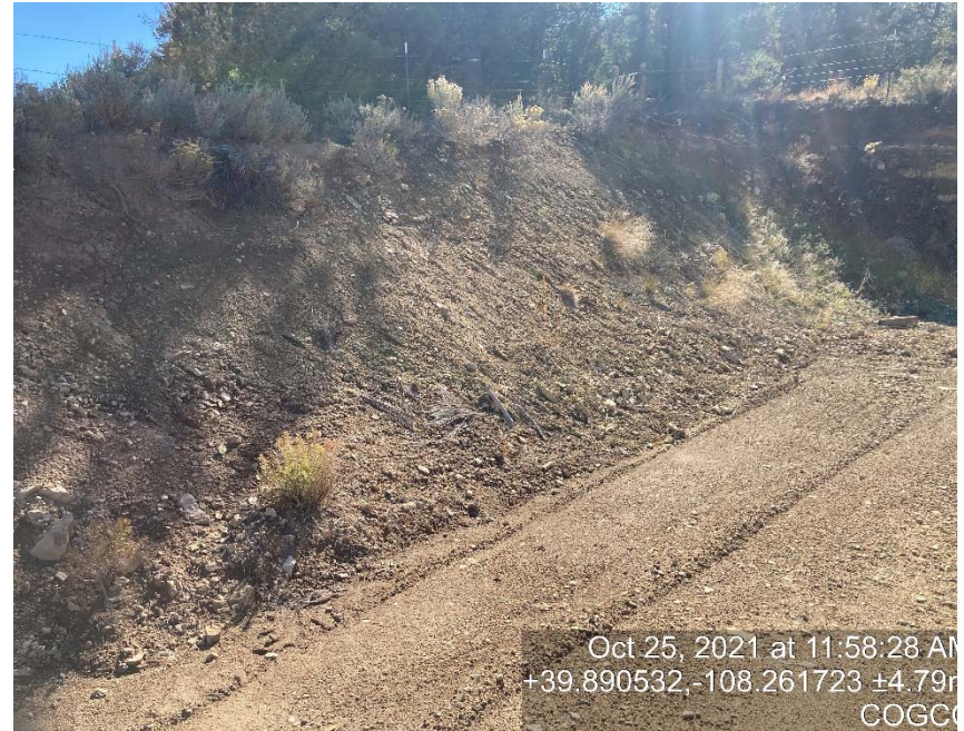
Lack of stabilization/erosion
