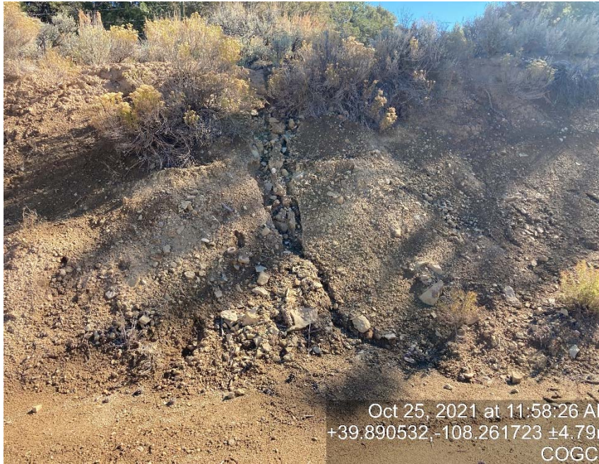
Lack of stabilization/erosion
