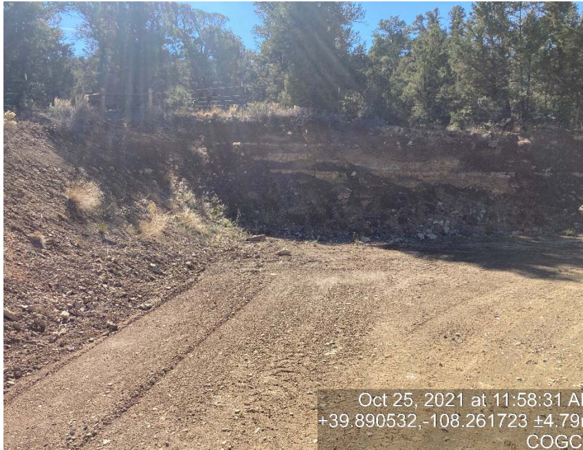
Lack of stabilization/erosion
