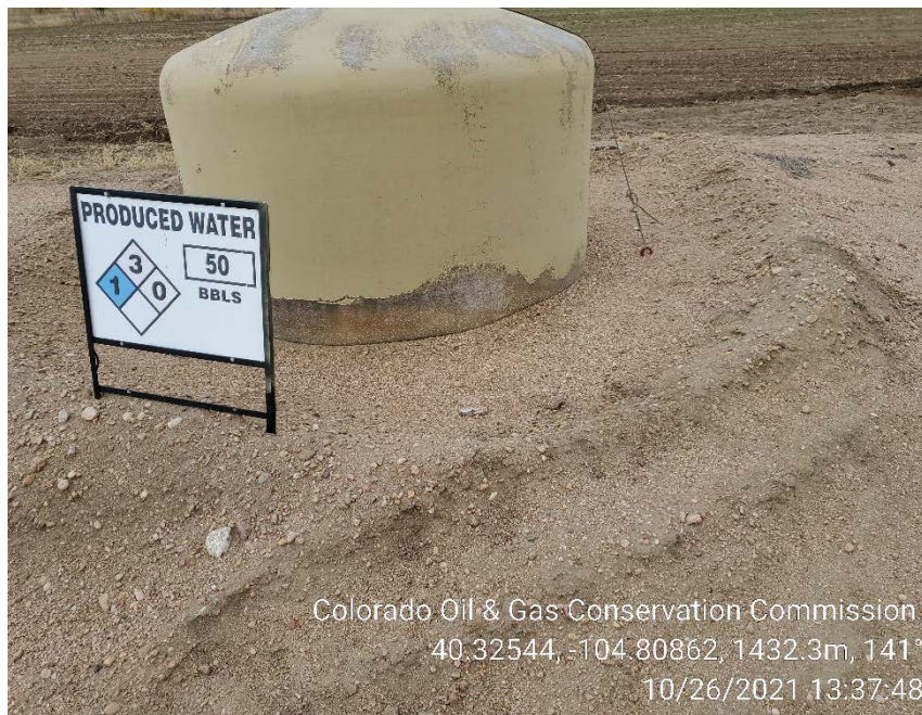
Produced water tank berm
