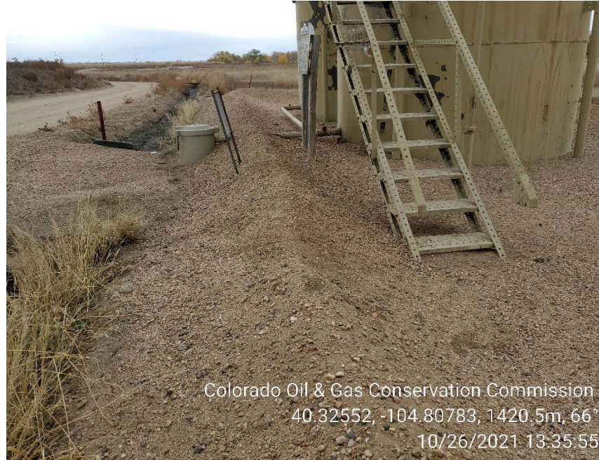
Crude oil tank berm
