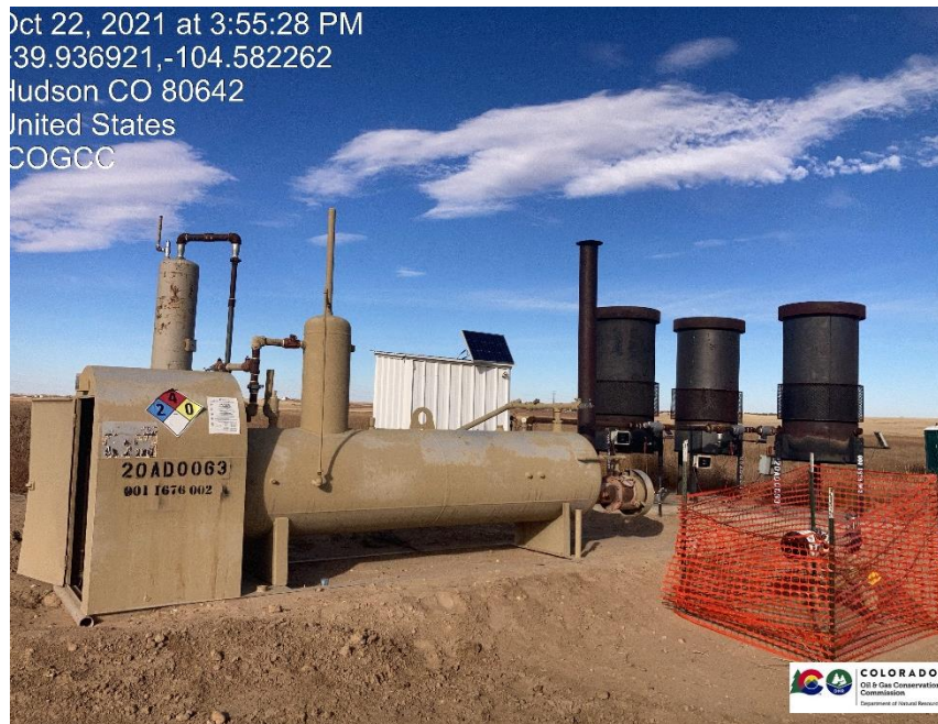
Pic 3 ECD used to Burn flare gas on location routed from gas meter run on location
