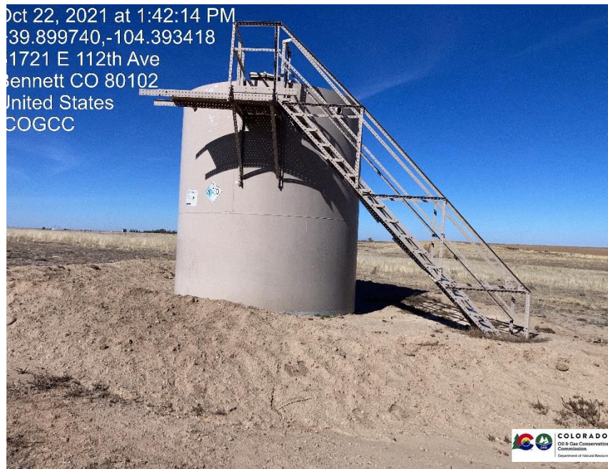
Pic 3 tank, berm needs to be rebuilt
