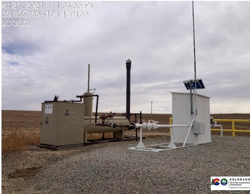
Pic 3 separator, and gas meter run.
