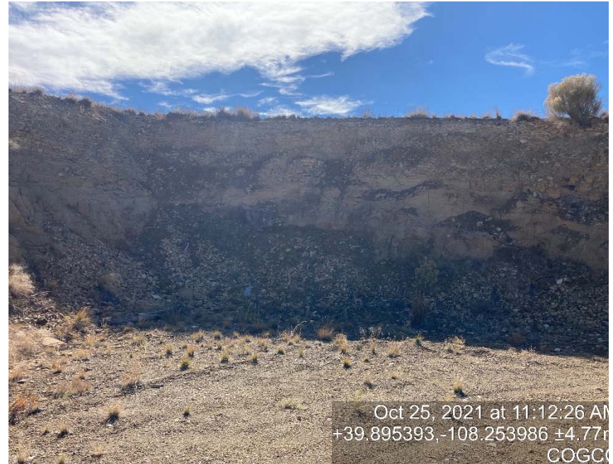
Lack of stabilization/erosion
