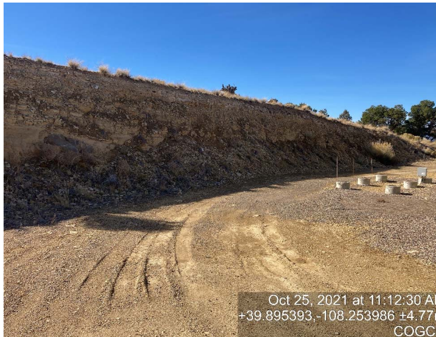
Lack of stabilization/erosion
