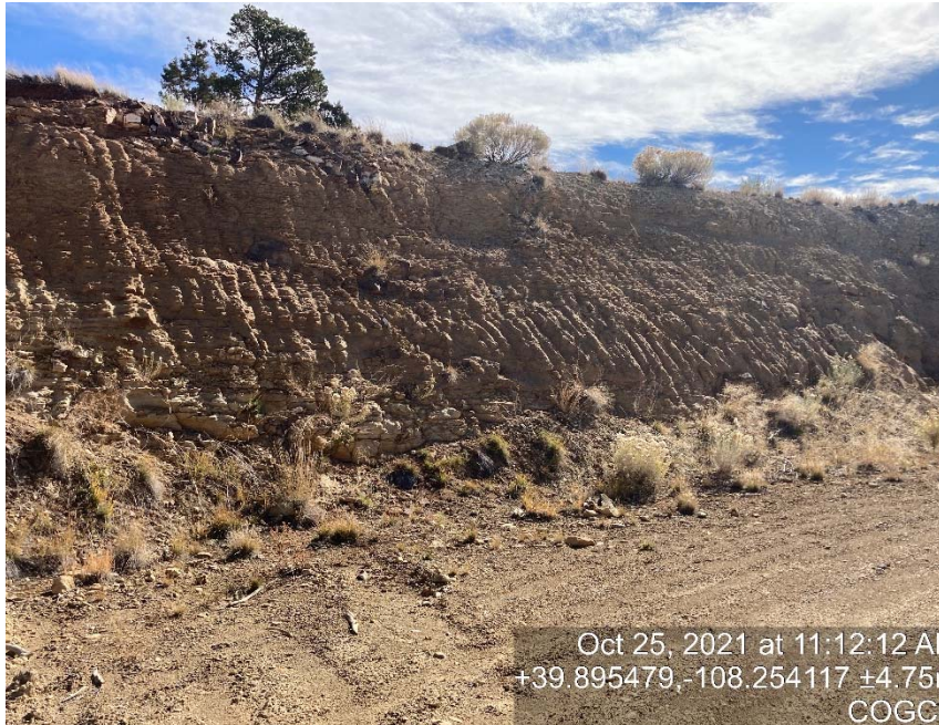
Lack of stabilization/erosion
