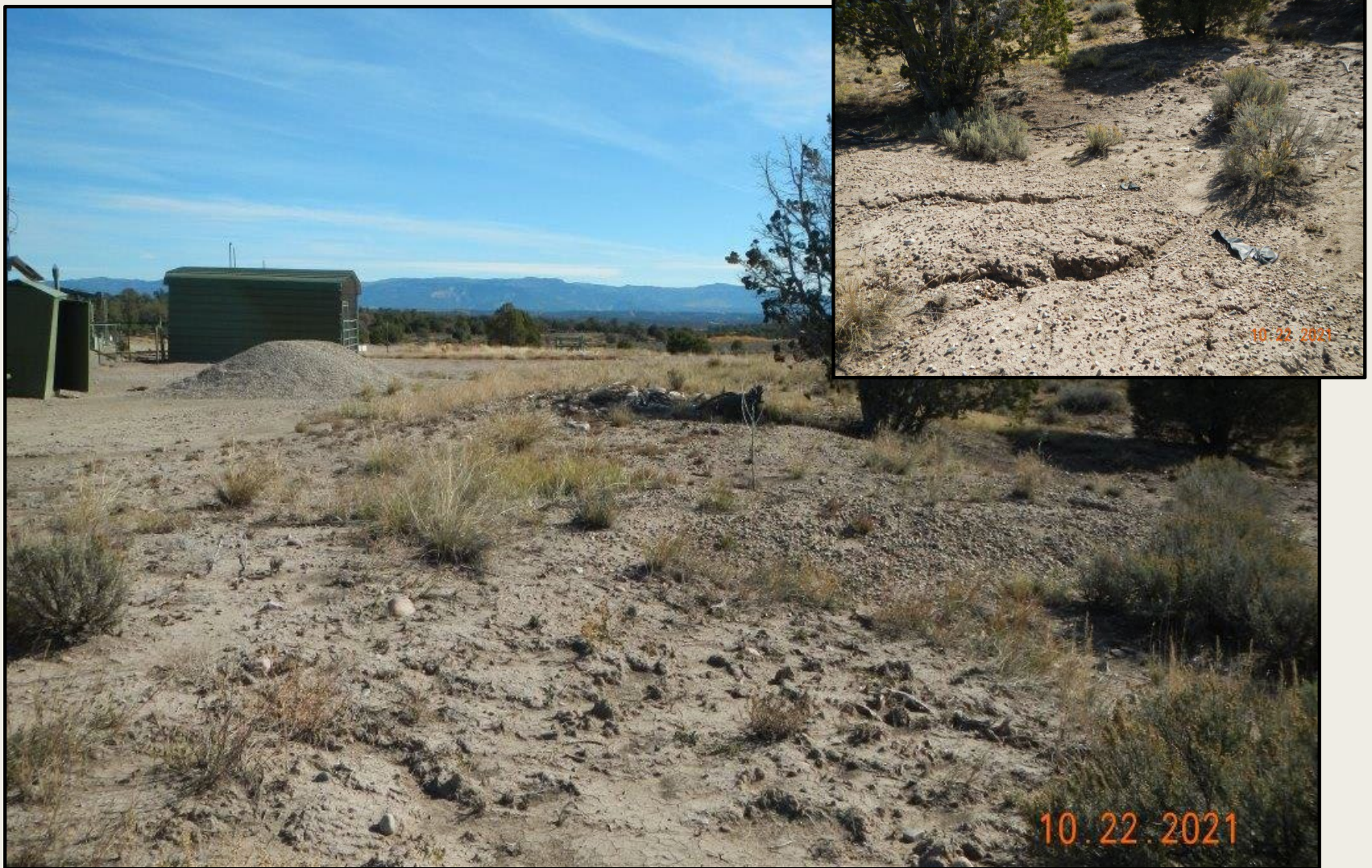
Photo 2. View of the southern project area from the southwestern corner facing eastward. Soils are not stabilized in this portion of the project area, with erosional channeling and sediment transport occurring. Inset shows an erosional channel approx. 12 in wide and deep in the southern fill slope.
