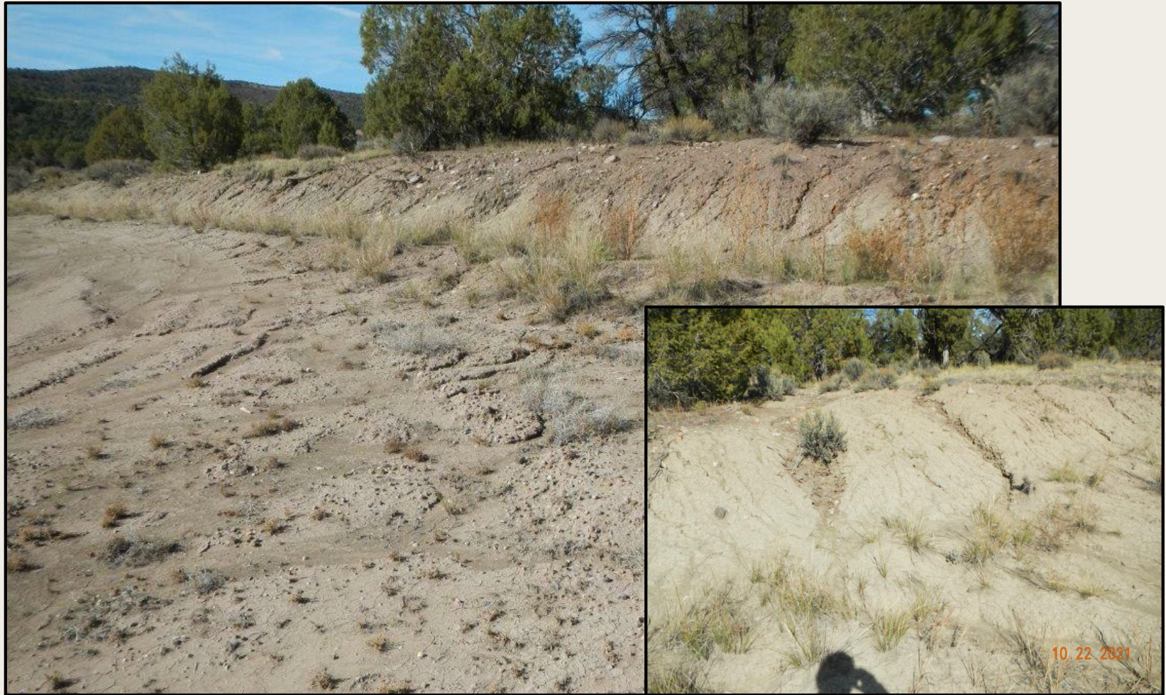
Photo 3. View of the northern cut slope. Multiple erosional channels and sediment deposition occurring. Inset shows more erosional channeling and sediment deposition on the well pad.
