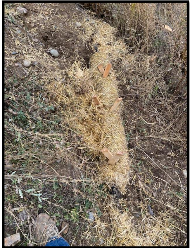
**Notes:** Waddles were installed in drainage area on south east of cut slope. Cattle got into waddles within 12 hours of installation. Petrox will monitor when cattle are moved out and will reinstall all stormwater and install mulch at that time.
