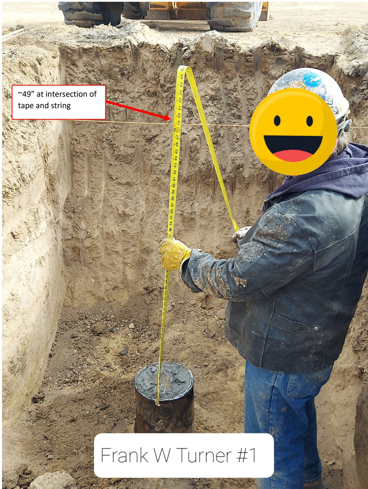
Photos showing the depth of cut for the well cap and the required information.
