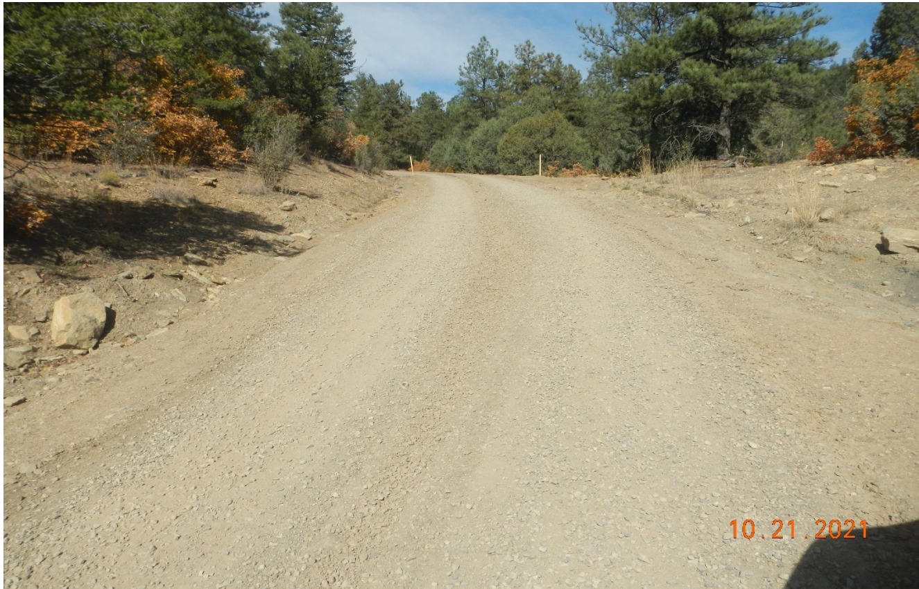
Photo 6. There has been road base spread on areas where vehicle rutting had occurred. The road has been regraded and repaired.
