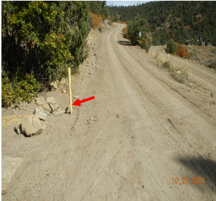
Photo 4. Facing north as the road ascends the hill side. A culvert has been installed at red arrow to properly divert stormwater away from the road.
