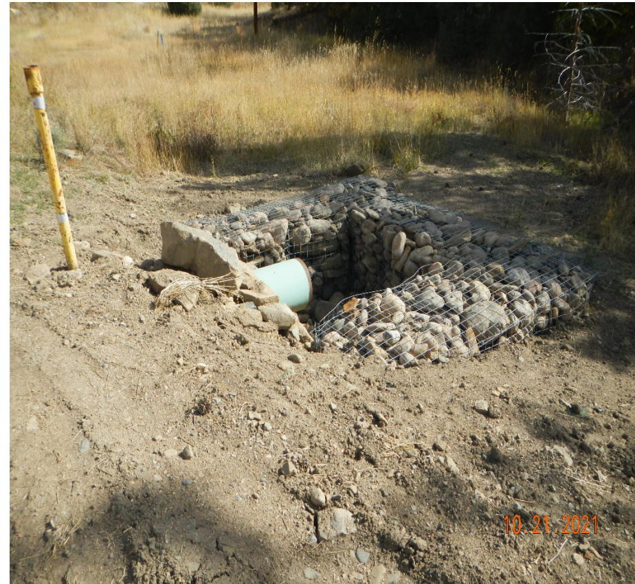
Photo 5. The culvert outlet gabion has been installed. This structure will need to be monitored and maintained to prevent sediment accumulation.
