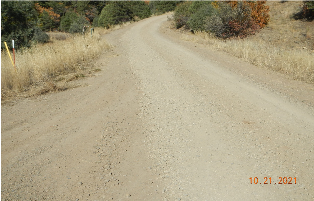
Photo 1. There has been road base spread on areas where vehicle rutting had occurred. The road has been regraded and repaired.
