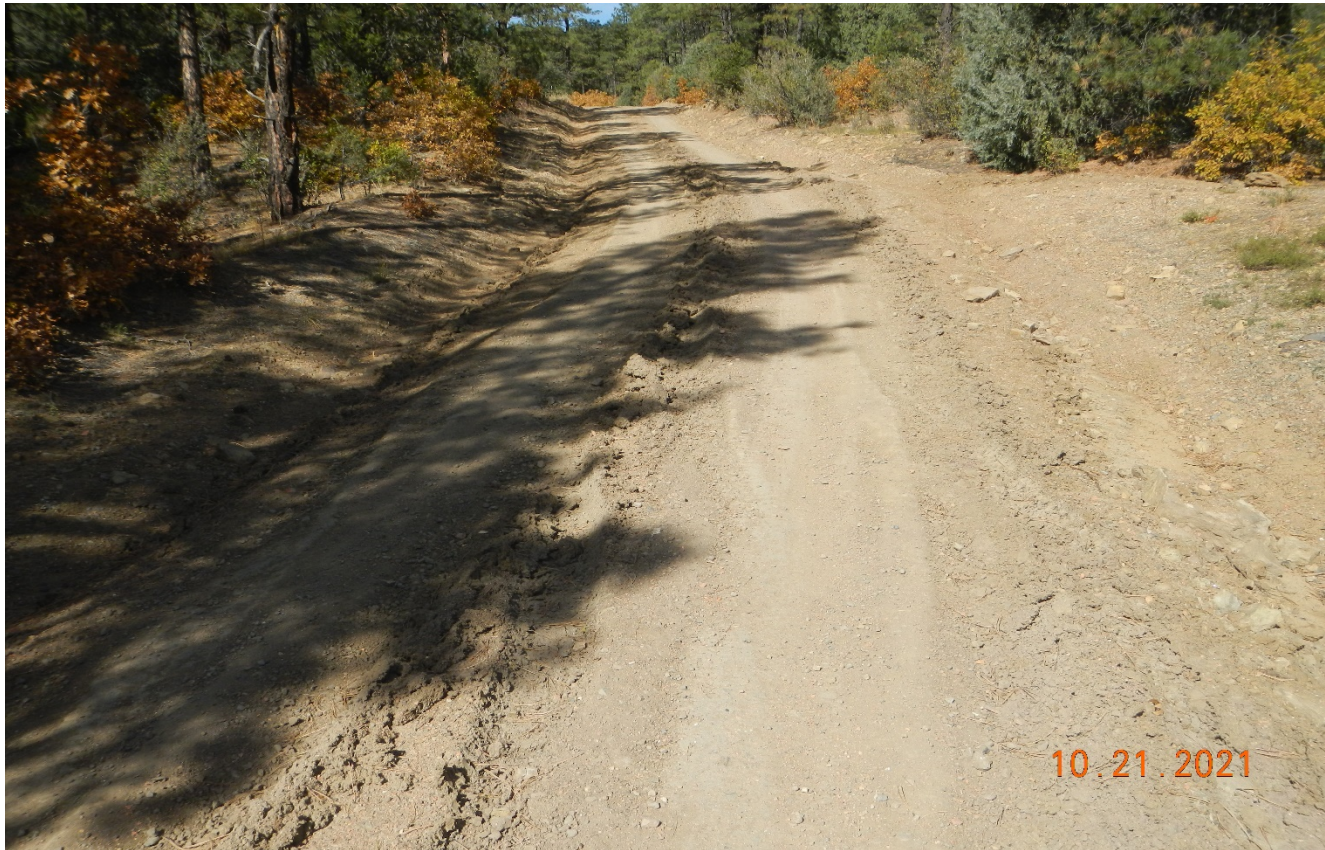
Photo 7. Facing northwest further along the road. There is vehicle rutting in this area which was not graveled. Additional gravel is needed in this area.
