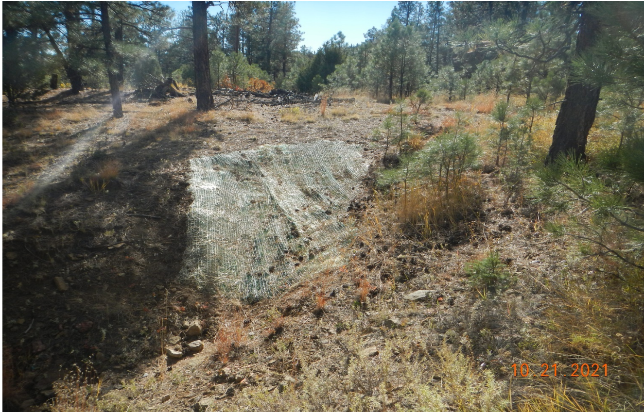
Photo 9. The area of erosion previously observed was repaired and stabilized with straw blanket.
