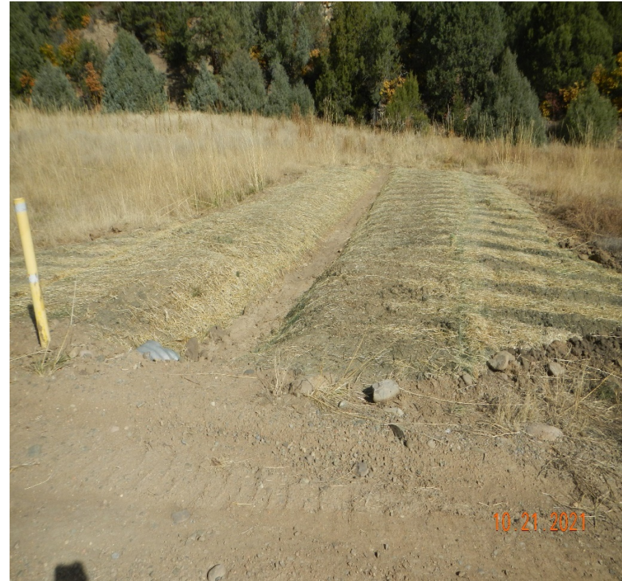
Photo 3. The culvert outlet has been repaired to allow stormwater diversion. Disturbance area was seeded and stabilized.
