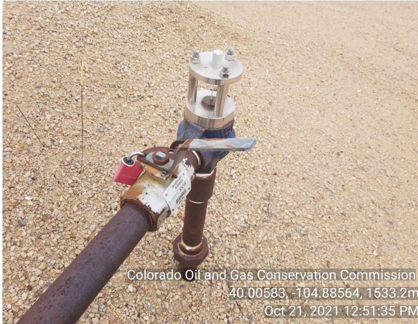
Photo 15 Gas sales line outlet from meter LOTO
