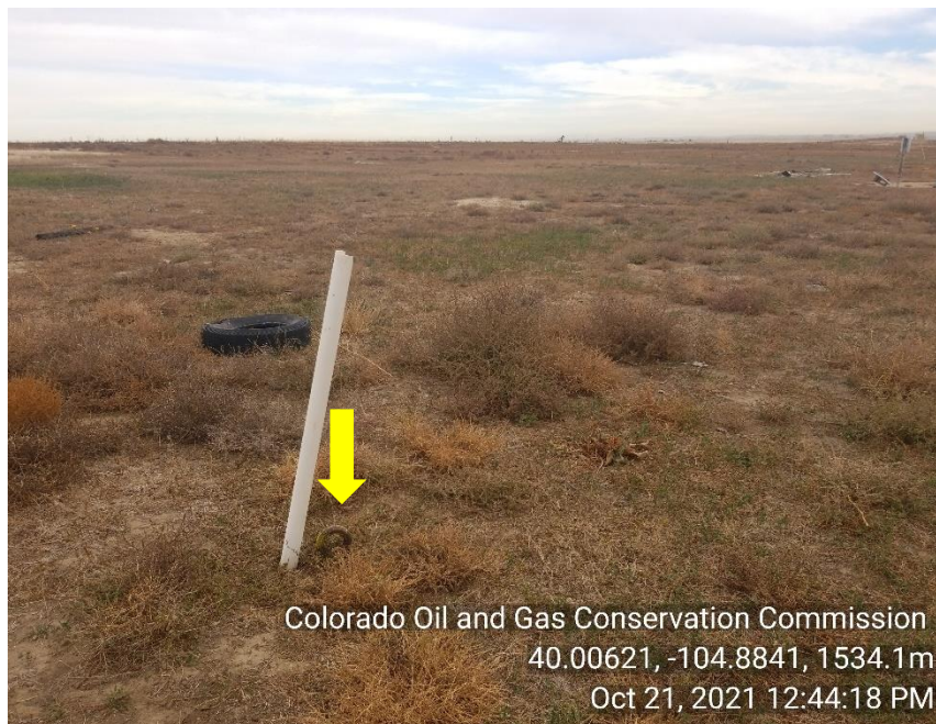
Photo 5 Guyline anchor not properly marked.
