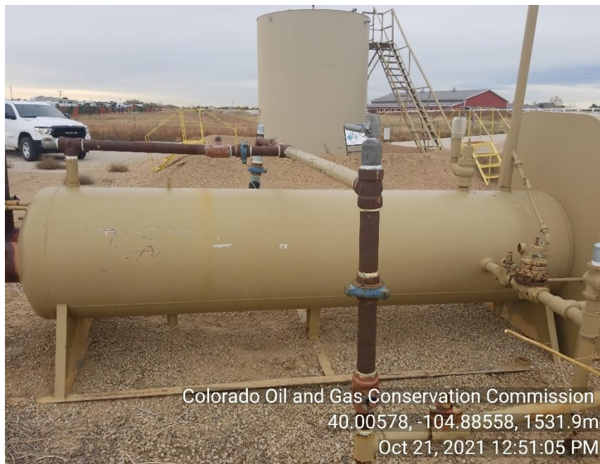
Photo 13 Supply line for HOZ Sep in closed position.
