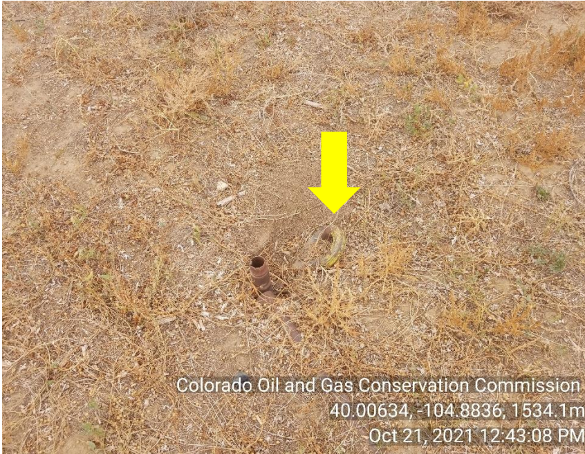
Photo 3 Guyline anchor not properly marked.
