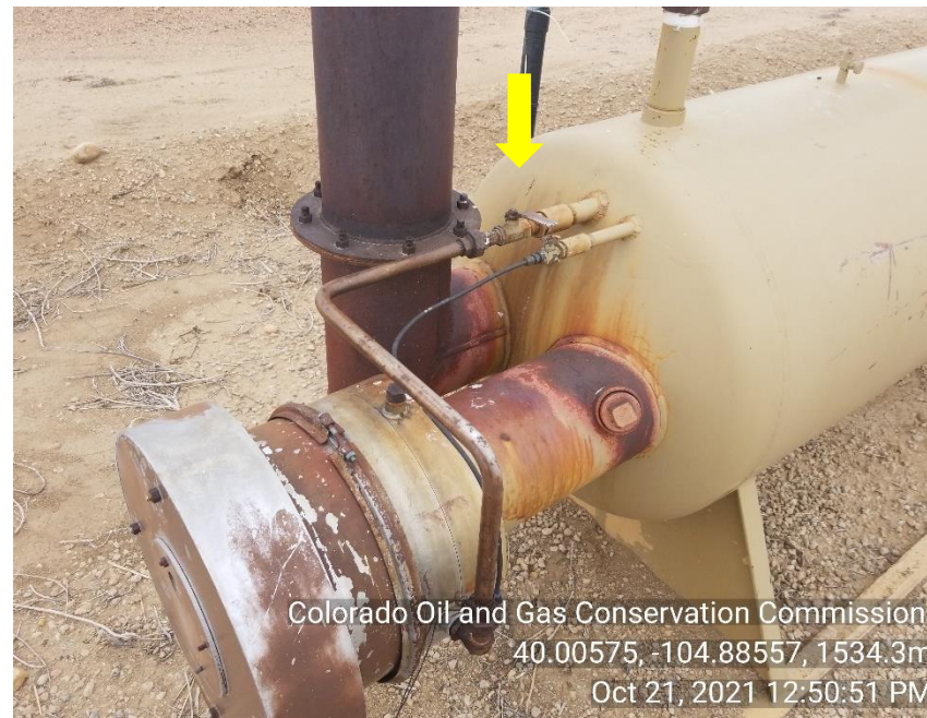
Photo 12 HOZ Sep not in use fuel gas line is in closed position.
