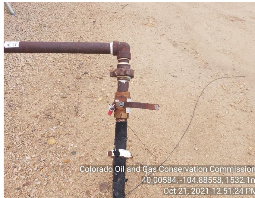
Photo 14 Gas sales inlet to meter is LOTO
