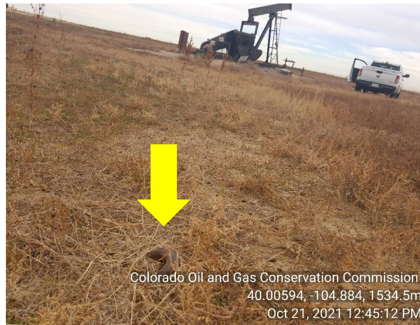
Photo 6 Guyline anchor not properly marked.
