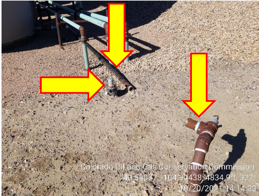
Photo 3 – Unmarked Risers and Unused Pipe
