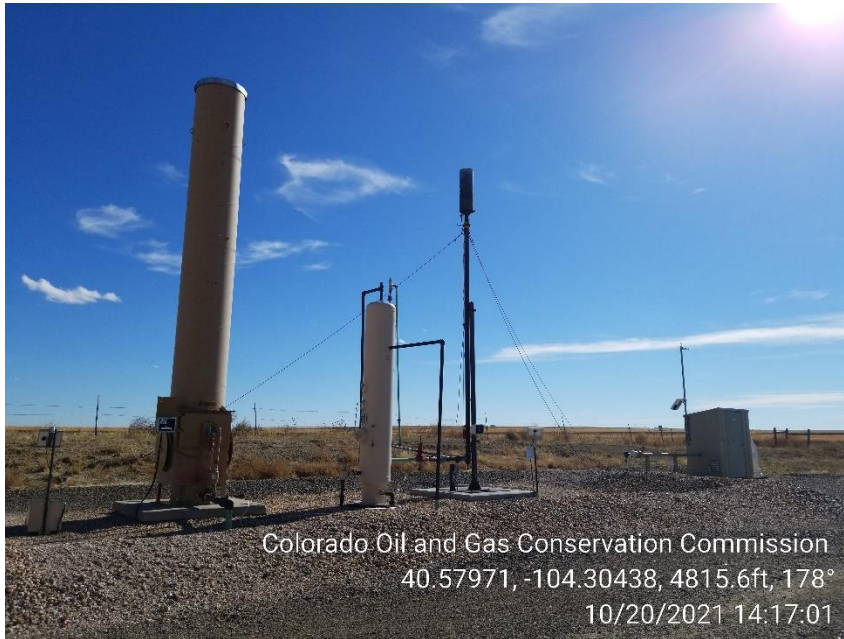
Photo 5 – ECD, Flare and Gas Meter
