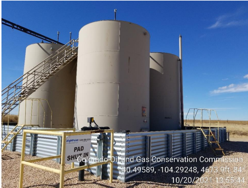
Photo 7 – Tank Battery
