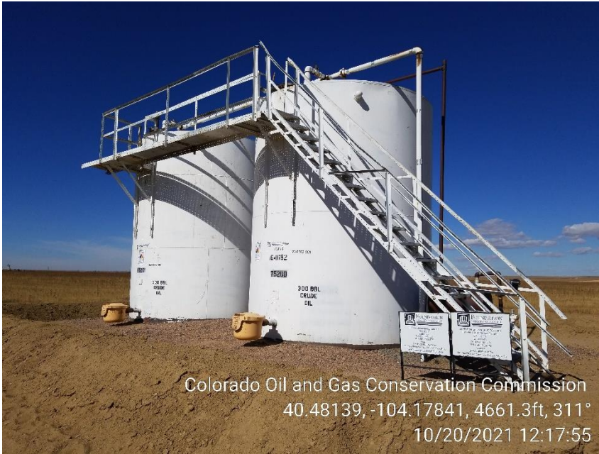
Photo 1 – Tank Battery
