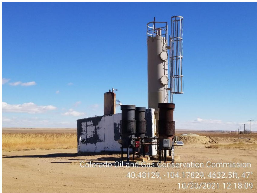
Photo 3 – Heater Treater and ECD
