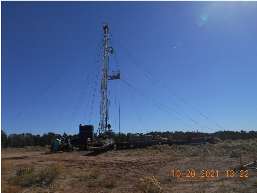
Rig on location for PA operations
