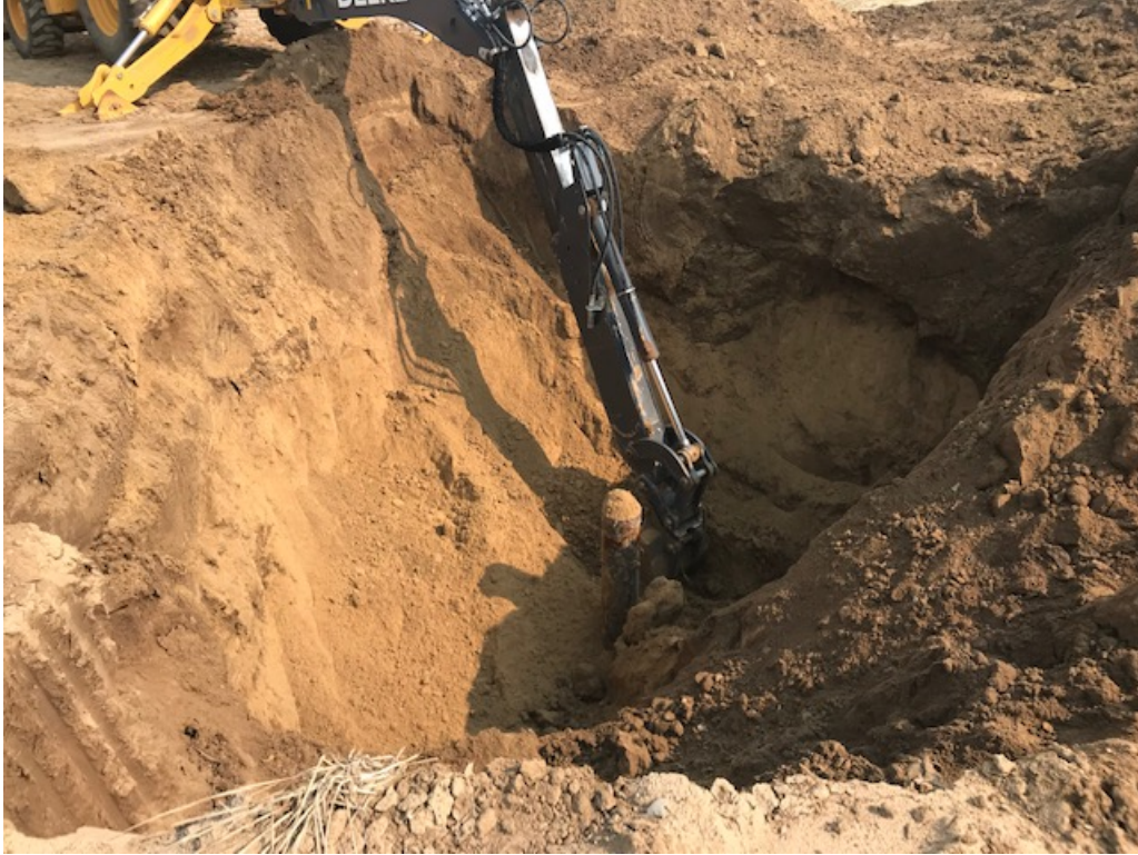
#3 - Looking Northwest at Wellhead Excavation; Marker Plate was knocked Off during Excavation
