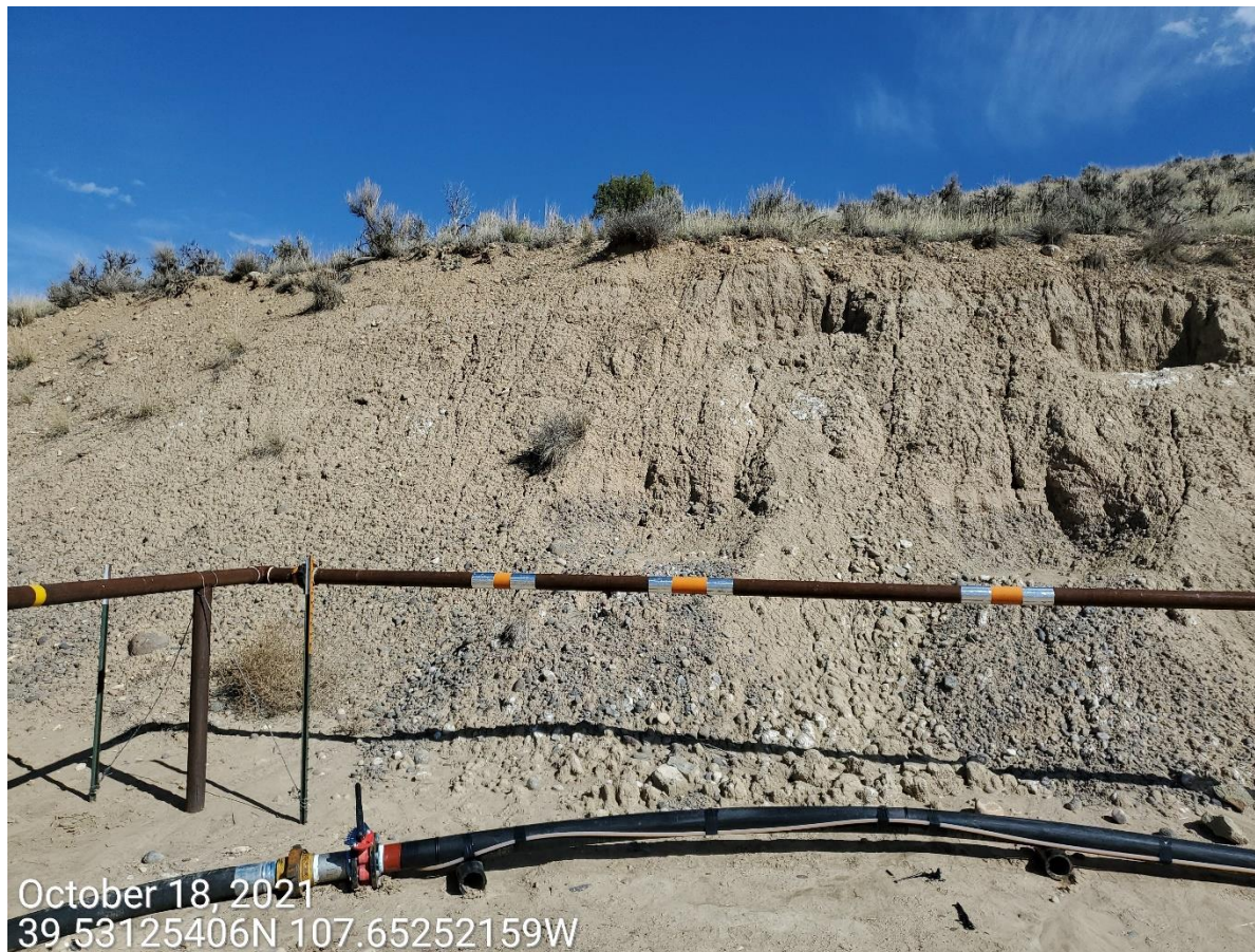
Photo 7: Photo shows example where control measures to protect and stabilize the slopes of the Location are missing or insufficient.
