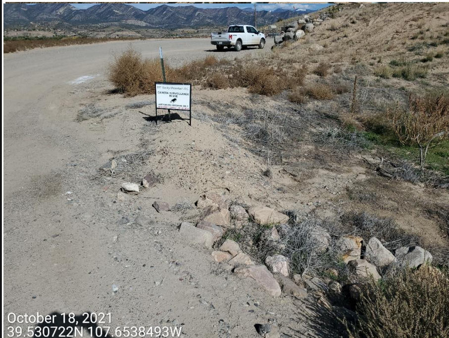
Photo 3: Photos taken from the Location entrance. Photo shows stormwater runoff from the Location resulting in sediment transport and deposition.
