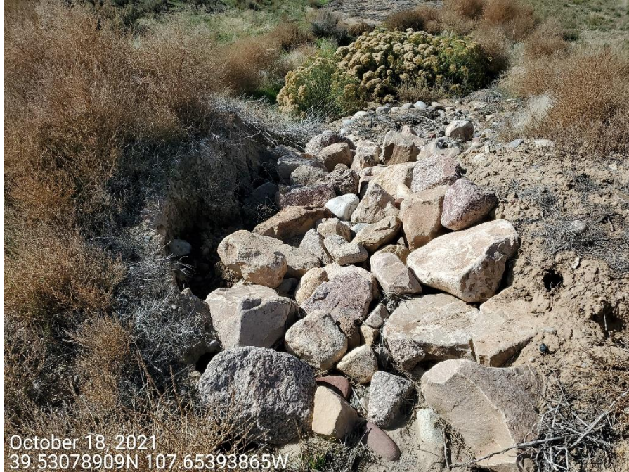
Photo 4: Photos taken from the outlet on the west end of the Location. Outlet has not been constructed in accordance with good engineering practices; use of geotextile under rip-rap not observed; stormwater runoff has resulted in degradation to both the BMP and offsite areas west of the Location.
