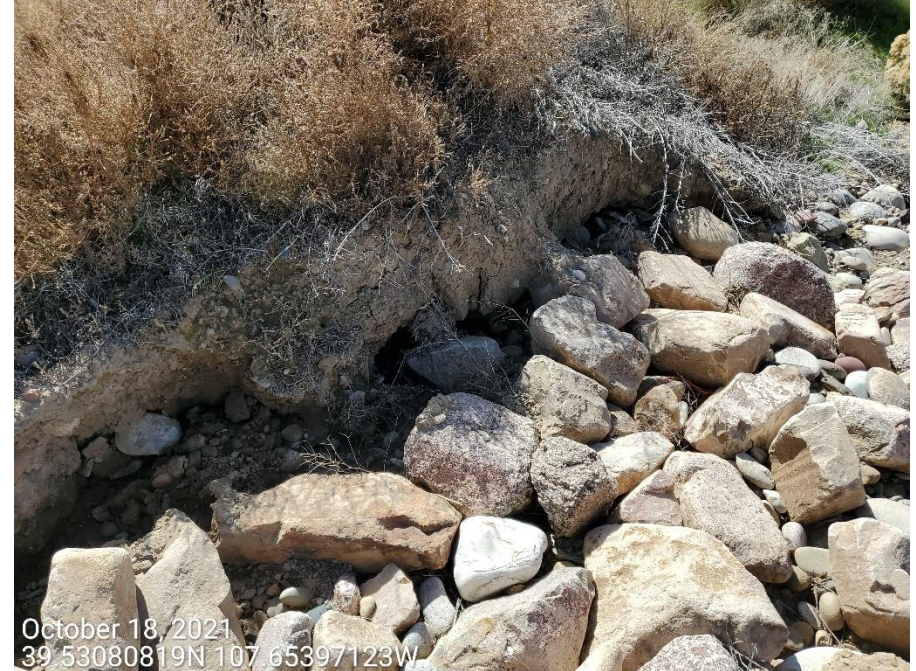
Photo 4: Photos taken from the outlet on the west end of the Location. Outlet has not been constructed in accordance with good engineering practices; use of geotextile under rip-rap not observed; stormwater runoff has resulted in degradation to both the BMP and offsite areas west of the Location.
