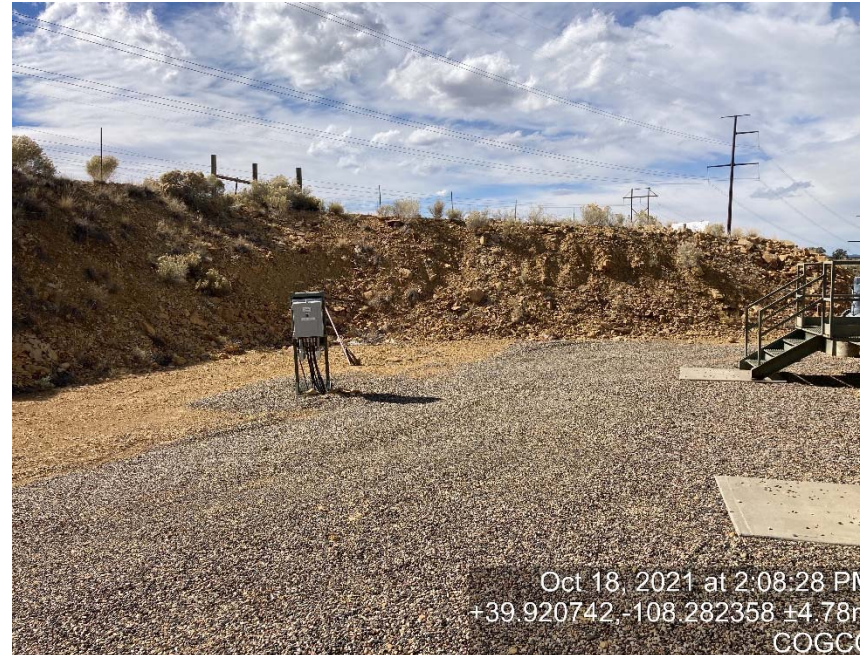
Cut slope shows signs of lack of stabilization
