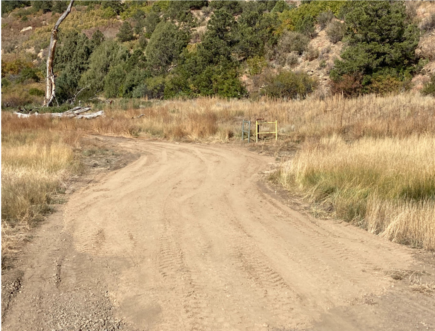
PHOTO 8: THE VEHICLE ACCESS TO THE DRIPS WERE STABILIZED WITH ROAD BASE.
