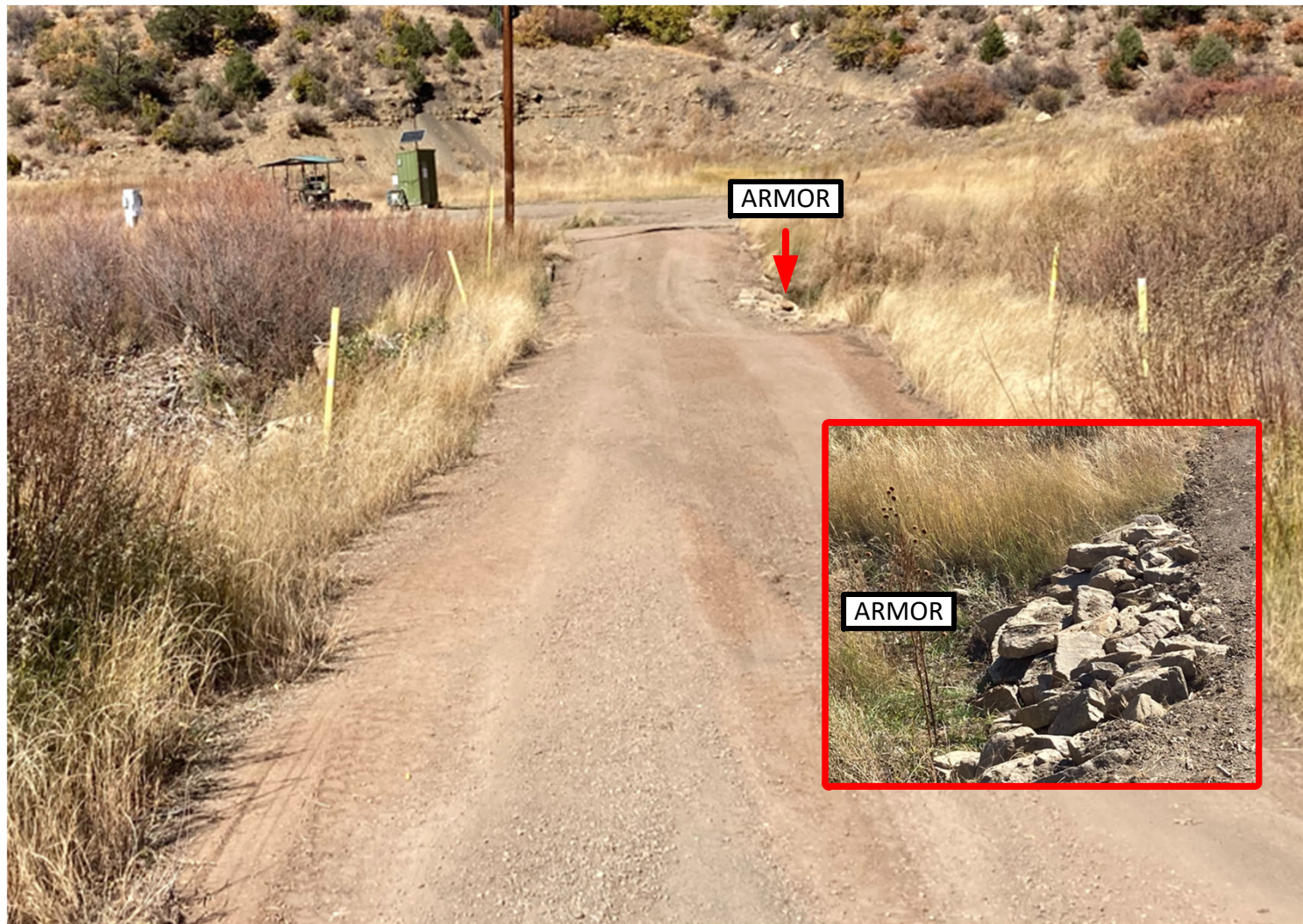
PHOTO 6: THE ACCESS ROAD TO LOCATION WAS REPAIRED WHERE WATER HAD SCOURED THE FILL PORTION OF THE ROADWAY. ARMOR WAS PLACED ON THE FILL FOR STABILIZATION. ADDITIONAL GRAVEL WAS INSTALLED ON THE ACCESS ROAD SURFACE.
