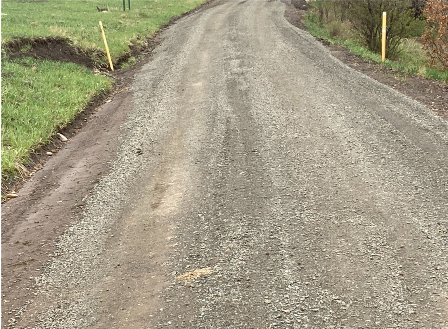
PHOTO 2: THE ROAD SURFACE WAS CROWNED TO CREATE SHEET FLOW AND ELIMINATE THE TIRE RUTS. RUN OFF IS DIVERTED TO THE CULVERT INLETS. ADDITIONAL GRAVEL WAS INSTALLED TO IMPROVE STABILIZATION.
