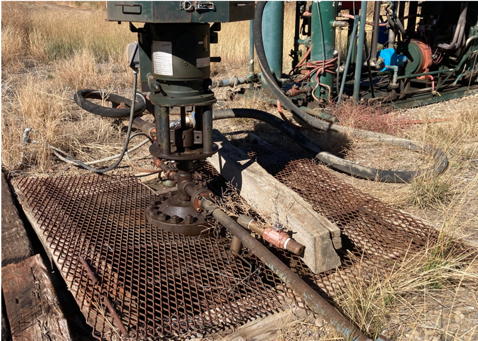
PHOTO 7: THE METAL GRATE WAS RECONFIGURED TO COVER THE CELLAR OPENING.
