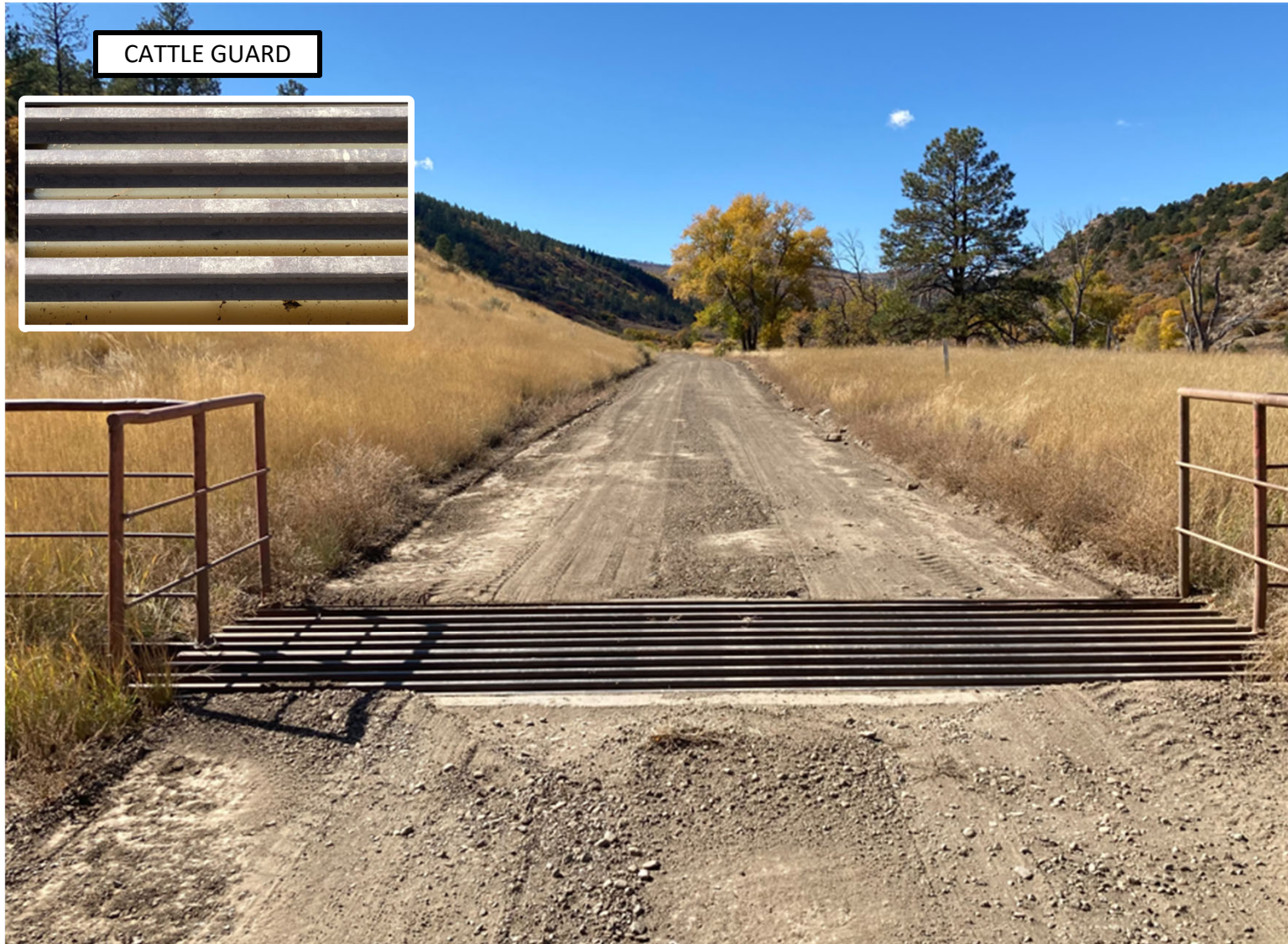
PHOTO 1: THE SEDIMENT WAS REMOVED FROM UNDERNEATH THE CATTLE GUARD.
