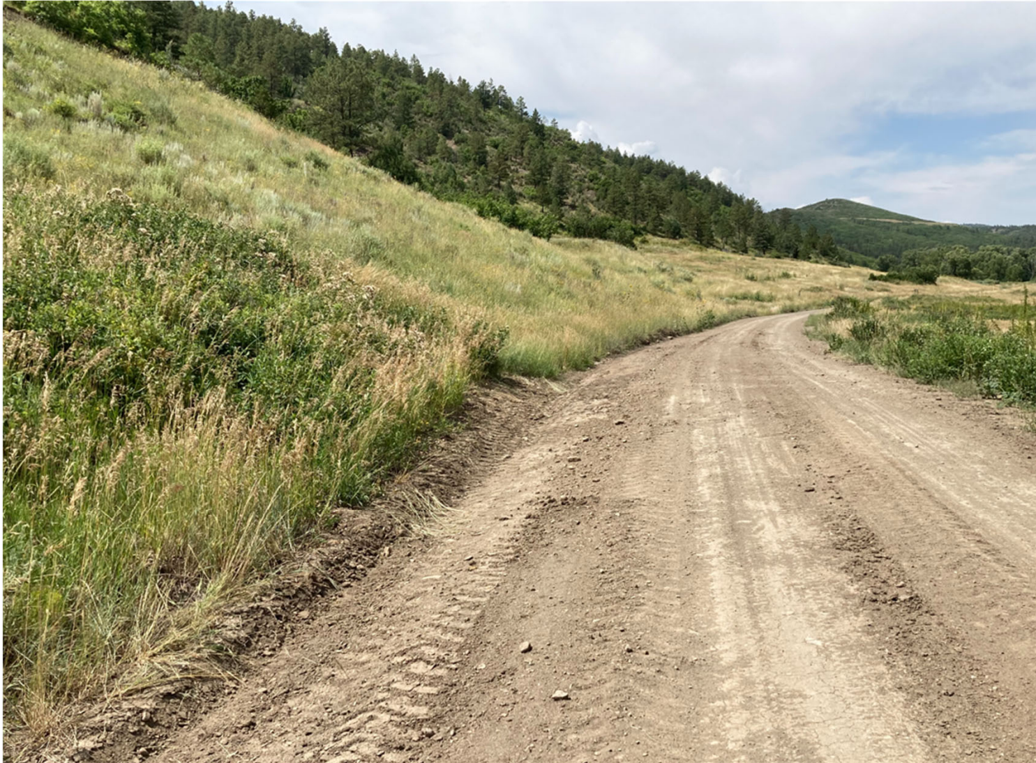
PHOTO 3: THE BAR DITCH WAS DOMINATED TO RECEIVE STORMWATER RUN OFF FROM THE ACCESS ROAD. THE ROAD SURFACE WAS CROWNED TO CREATE SHEET FLOW AND ELIMINATE THE TIRE RUTS.
