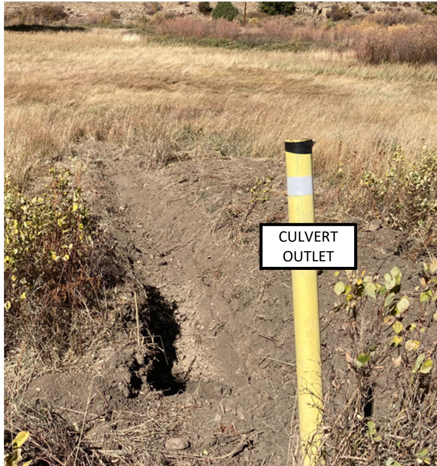
PHOTO 5: SOME OF THE CULVERT OUTLETS ALONG THE MAIN SOUTH FORK LEASE ROAD WERE BELOW GRADE AND WOULD NOT DRAIN PROPERLY. DRAINAGE WAS ESTABLISHED FOR THE OUTLETS. THE CULVERTS WERE CLEANED OUT WITH THE HYDRO-VAC EQUIPMENT AND THE SEDIMENT ACCUMULATION WAS REMOVED FROM THE CULVERT INLETS.
