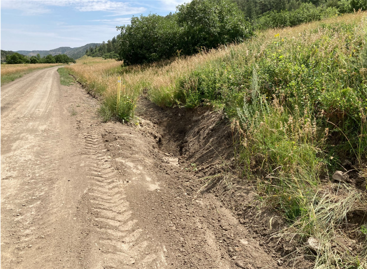
PHOTO 4: THE SEDIMENT ACCUMULATION WAS REMOVED FROM THE BAR DITCH. THE BAR DITCH WAS DOMINATED TO RECEIVE STORMWATER RUN OFF FROM THE ACCESS ROAD. THE ROAD SURFACE WAS CROWNED TO CREATE SHEET FLOW AND ELIMINATE THE TIRE RUTS.
