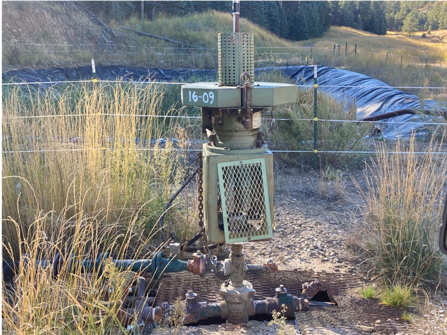
PHOTO 1: THE WELLHEAD PACKINGS WERE REPLACED TO STOP THE WATER LEAK. NO IMPACTS WERE DISCOVERED.
