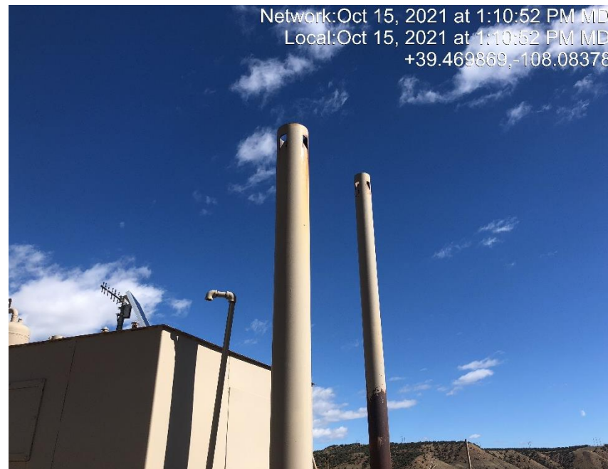
Photo #5091 Bird protectors missing on separator burners.
