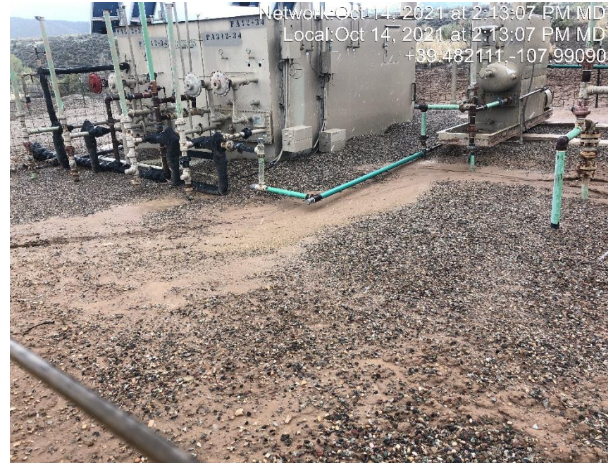
Photo #5087 Sediment encroaching on equipment.
