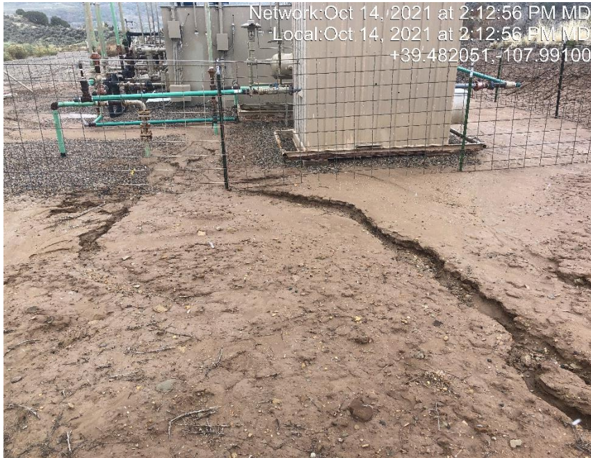
Photo #5086 Rill erosion occurring on location.
