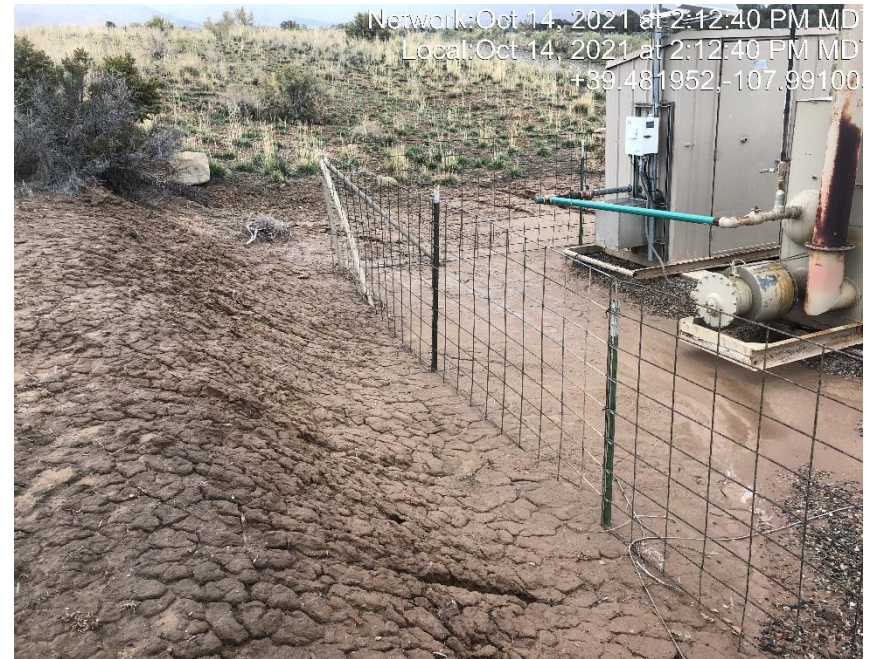
Photo #5085 Run on to location is not being controlled.
