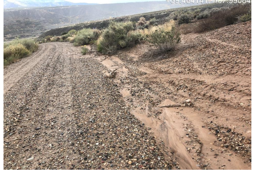
Photo #5079 insufficient velocity checks in ditch.
