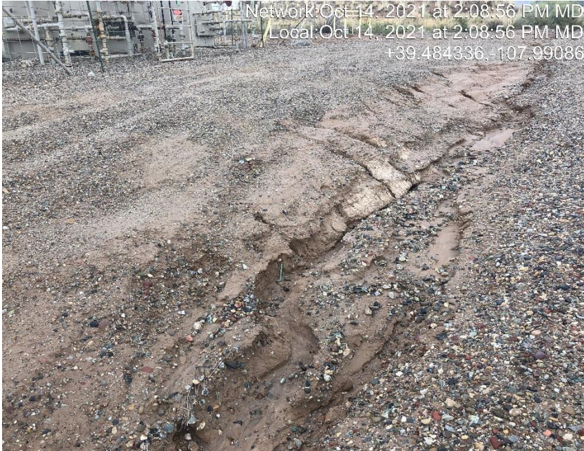
Photo #5081 Rill erosion occurring in ditch.
