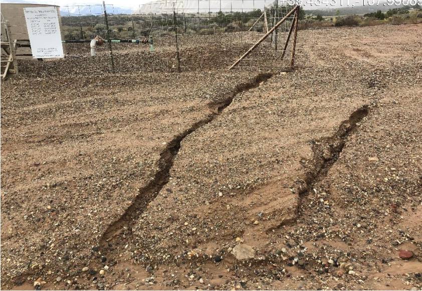
Photo #5078 Rill erosion occurring on location.
