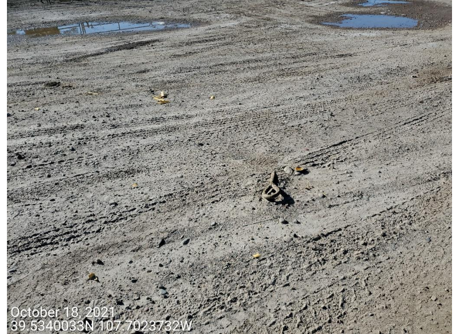
Photo 8: Photo shows example of anchors observed on the Location not properly marked.
