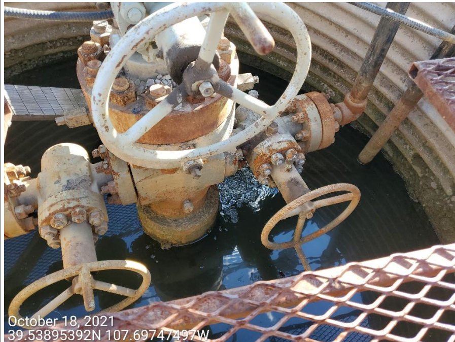
Photo 9: Photos show gas observed leaking from the A4 and A1 wells.
