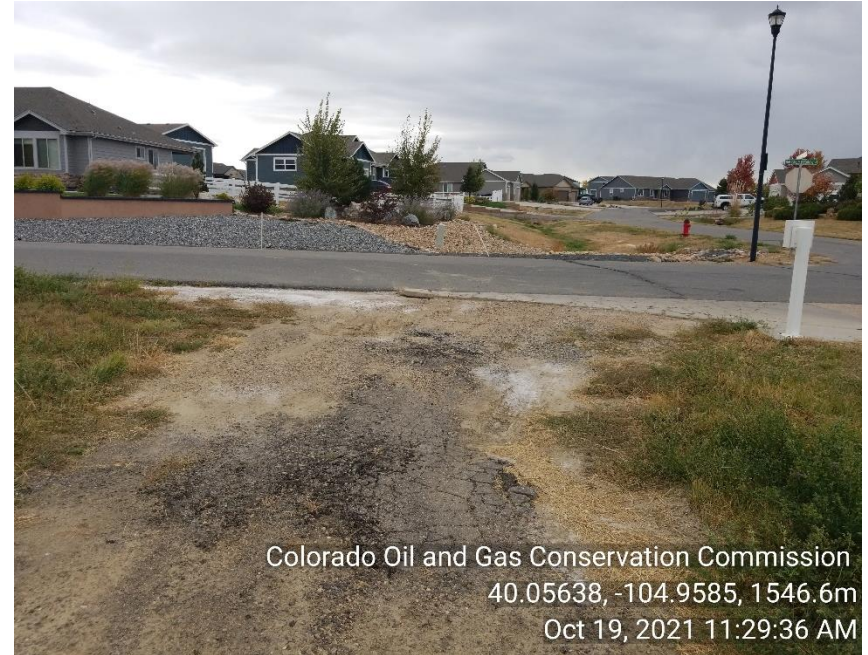
Photo 2 Tracking pad not maintained
