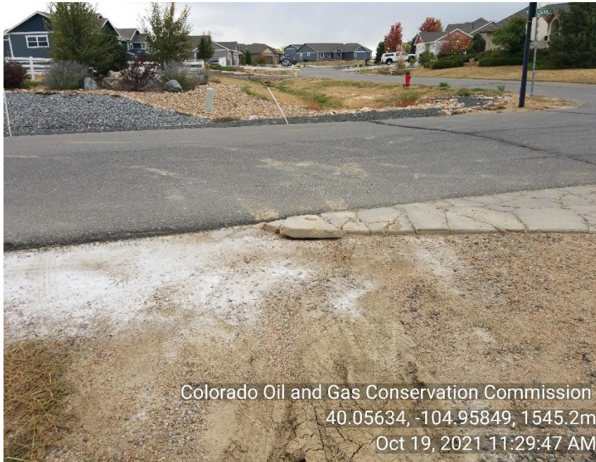
Photo 3 Sediment being carried onto public road.
