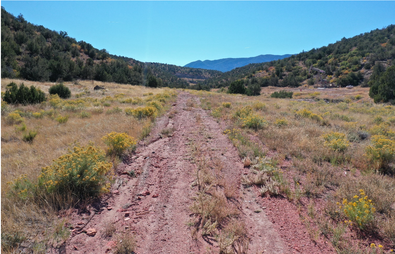
Photo 2. Facing south along the access road. Erosion along the road has gotten worse since previous inspection.
