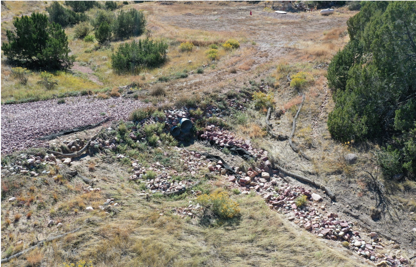
Photo 4. The outlet of the stream crossing has eroded and washed out. There are wattles, liner and rock rip/rap that are now displaced into the stream bed. This area needs to be repaired immediately.
